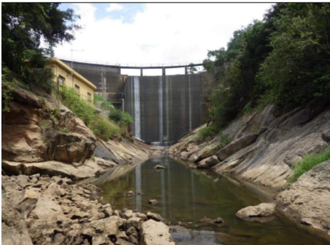
Photo 2: Flow Regulation, Channel and bed modification (A2; February 2018)
