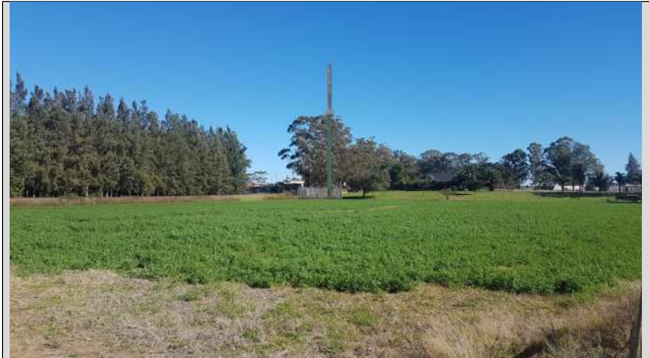
Figure 5: Visual Impression of a Monopole Mast (Please note this impression is not for Portion 87 of the Farm No. 23)
