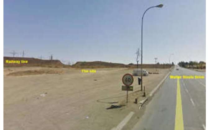
Figure 5: View of the railway line west of the site
