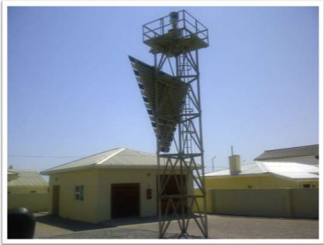
Figure 7-2 Existing lattice, aluminium lighthouse structure.
