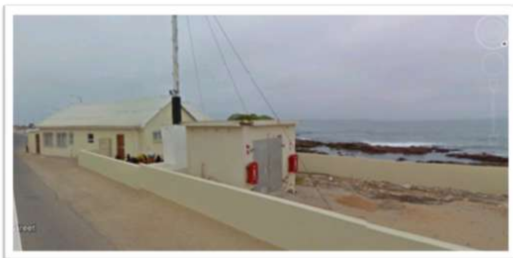
Figure 4 View of the structure from north to south.
