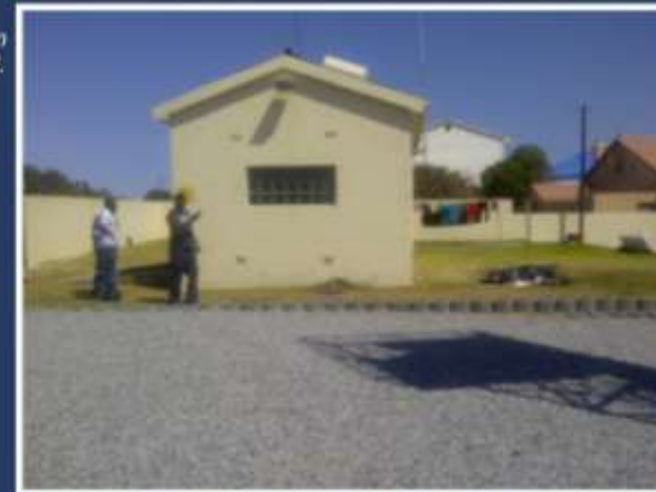
Figure 4: View of the existing engine room on ERF 45 which will connect to the new lighthouse.
