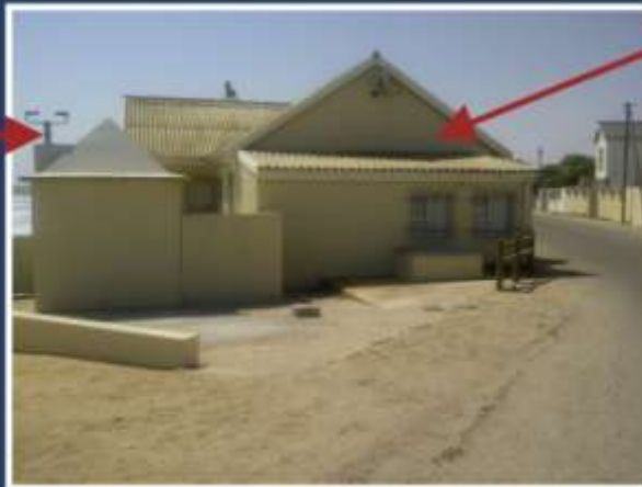
Figure 3: View of the site with the lean-to structure that will be demolished.
