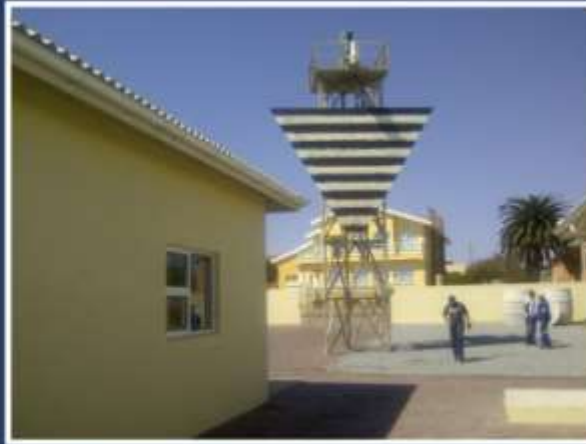
Figure 1: Front view of the existing lighthouse from Beach Street. This lighthouse will be decommissioned.
