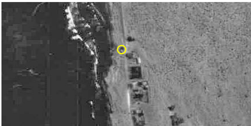
Figure 3 Excerpt from 1937 aerial photograph indicating the magazine. This is the only structure visible on the western side of Beach Street.
