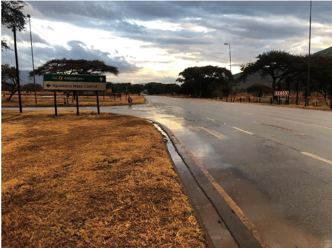
Figure 4. Weighbridge turnoff from the N4 toward the Macrodump general fill stockpile area.
