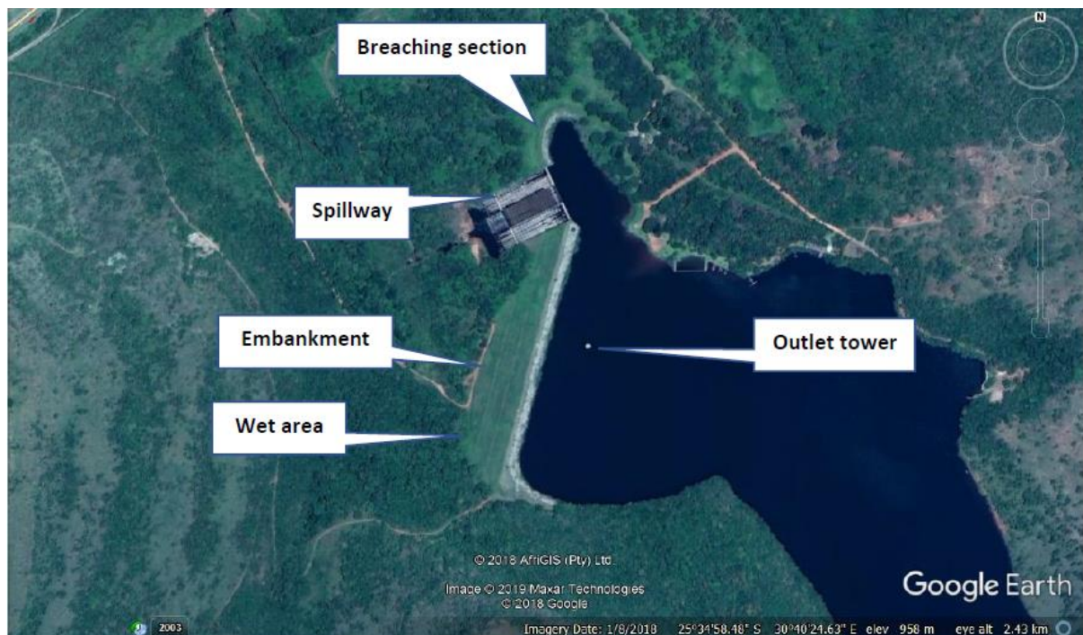
Figure 22. Areas of concern on the Ngodwana Dam wall, for which remedial work will be required.
