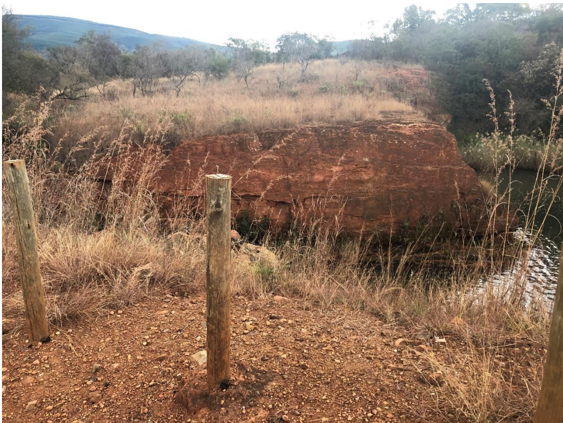
Figure 17. Location of footbridge over the Ngodwana River beneath the spillway, which will create pedestrian access to both sides of the dam wall.
