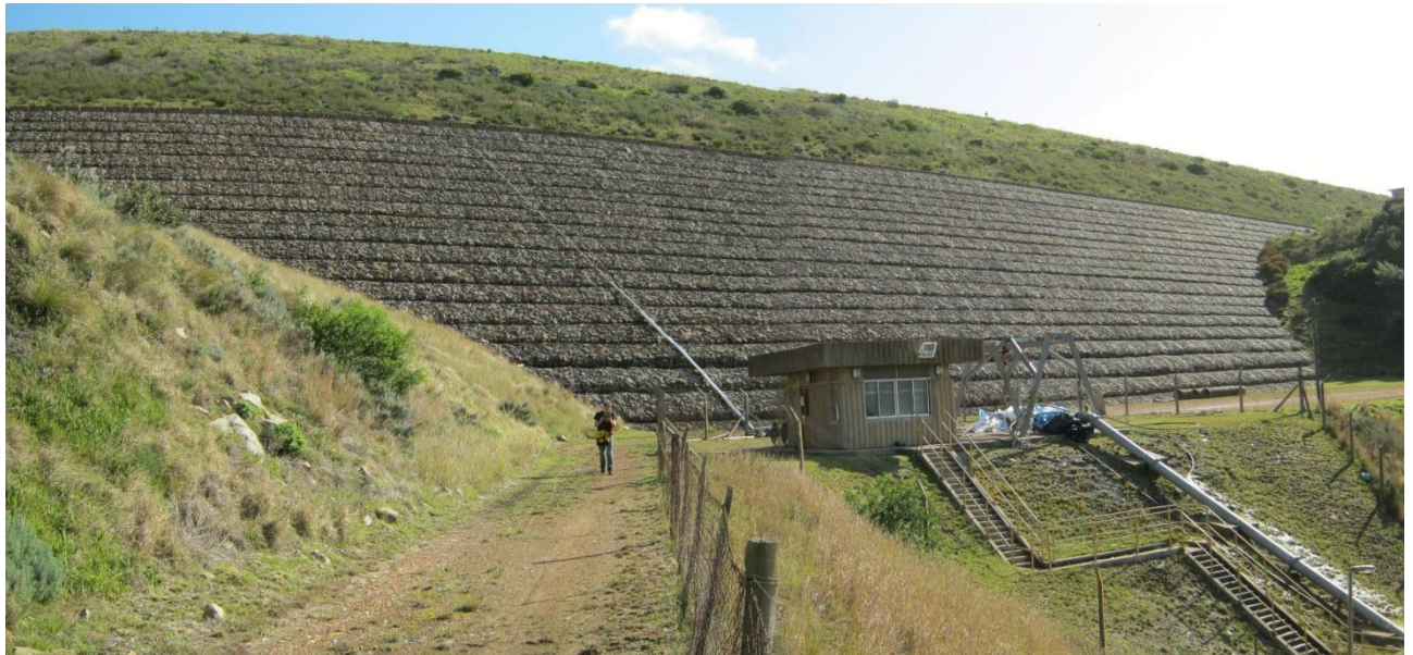
Figure 19. Reinforced rockfill used at Impofu Dam.
