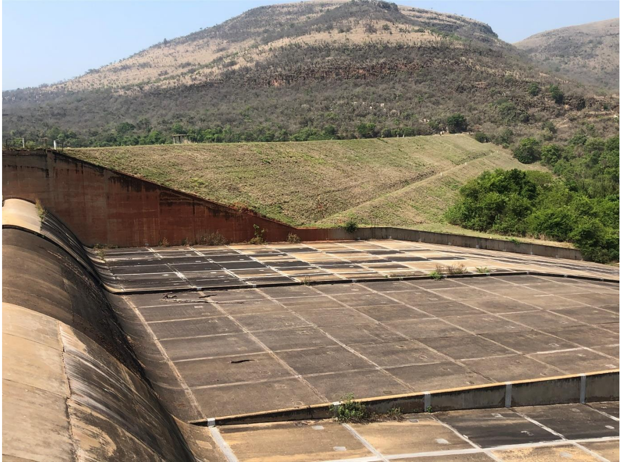
Photograph 4. The concrete spillway and main embankment.
