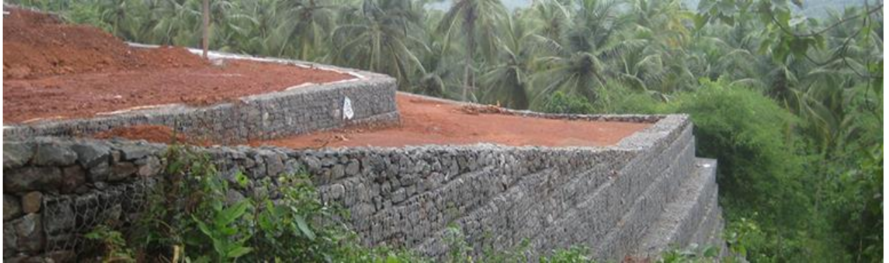
Figure 20: Gabion retaining wall.
