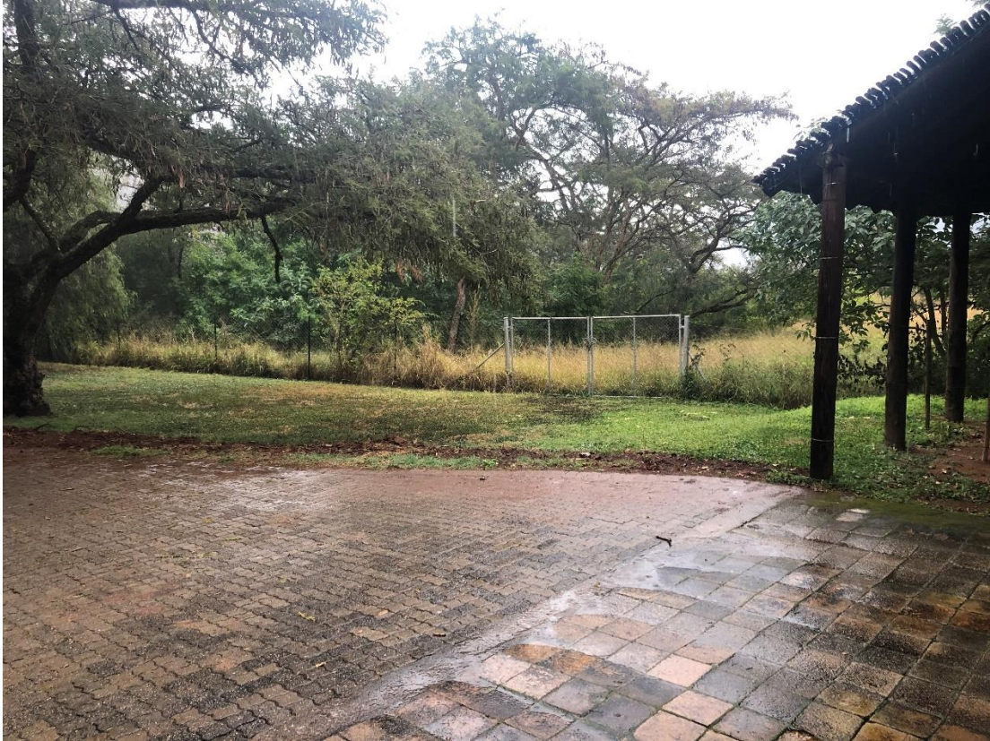
Figure 8. Current access gate to the right flank of the Ngodwana Club entrance.
