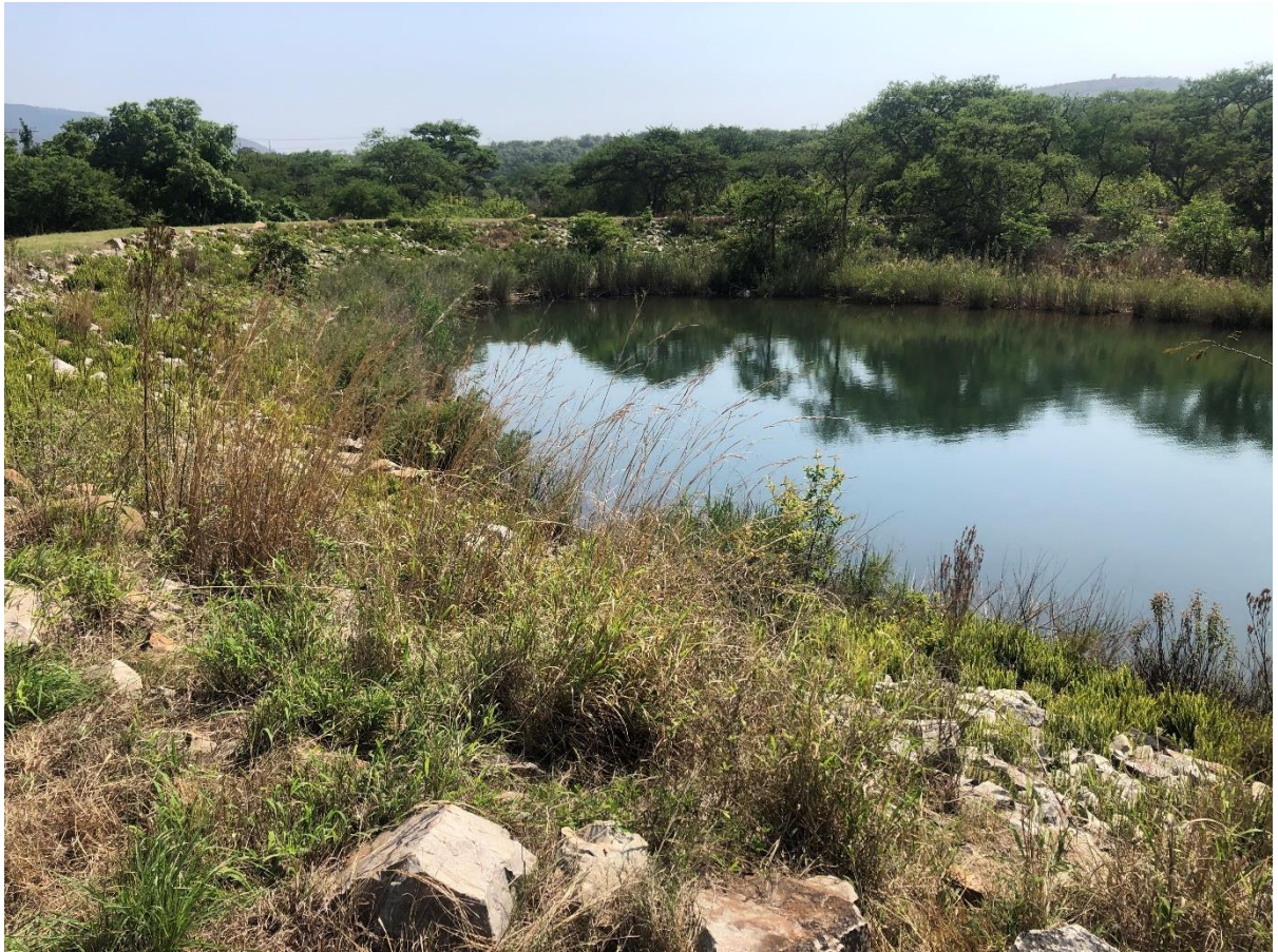
Photograph 3. The right flank (fuseplug) embankment.
