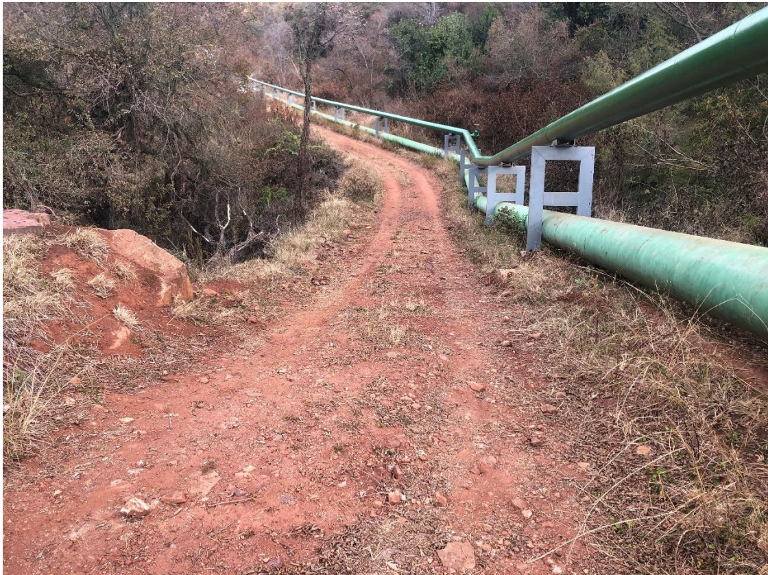
Figure 16. Existing gravel access road running from the WTW along the raw water pipeline to the main dam embankment.
