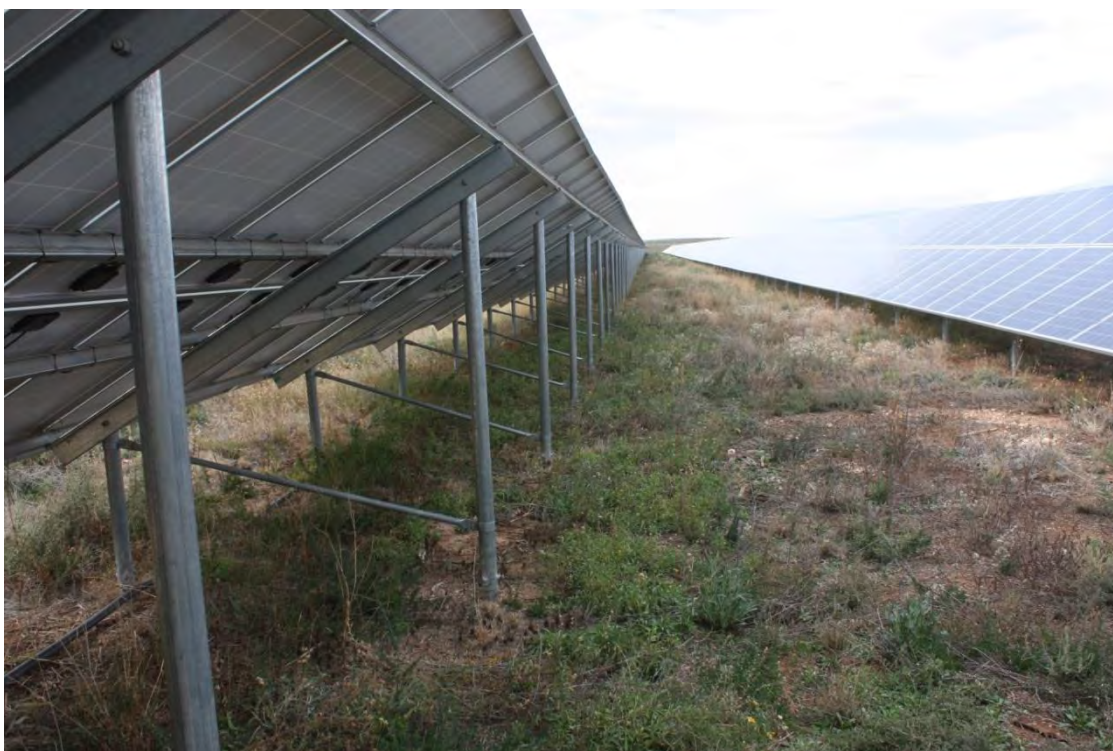
Figure 7.8: Image of solar arrays indicating the limited influence that such structures generally have on the flow of surface waters within a solar facility.
