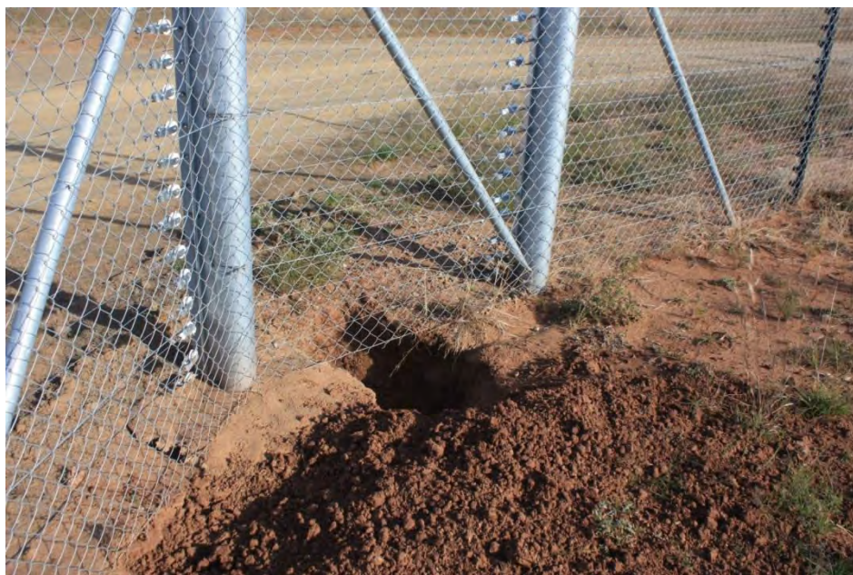
Figure 7.11: Fossorial movement under fences by larger animals, porcupines and Aardvark ( Orycteropus afer ).
