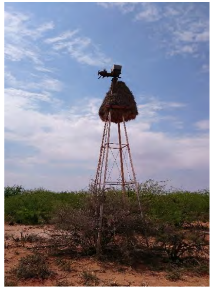
BH8 - wind pump
