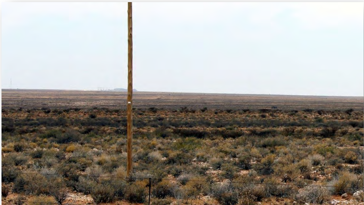
Figure 8.13: View from photo site SCA014 eastwards. The tower at Rugseer Siding is visible on the left and the new substation more towards the centre.
