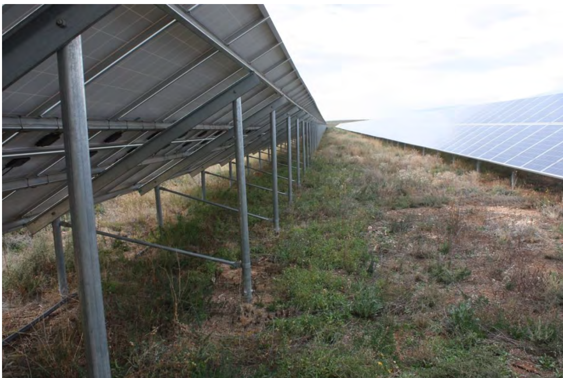
Figure 7.9: Image of solar arrays indicating the limited influence that such structures generally have on the flow of surface waters within a solar facility.
