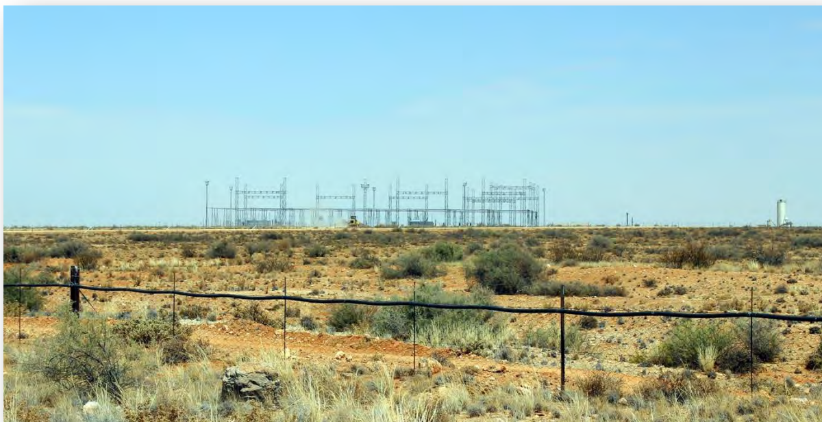
Figure 8.14: Nieuwehoop Substation currently under construction (Photo site SCA010)
