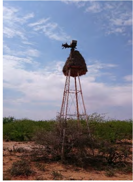
BH8 - wind pump
