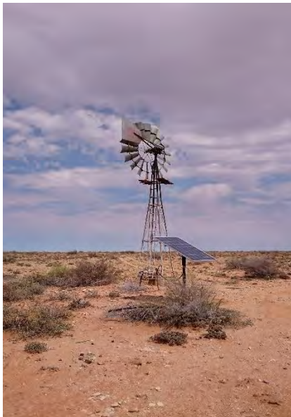
BH5 - wind pump
