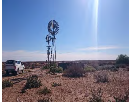
BH2 - wind pump
