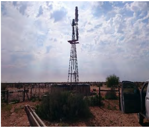
BH3 - wind pump
