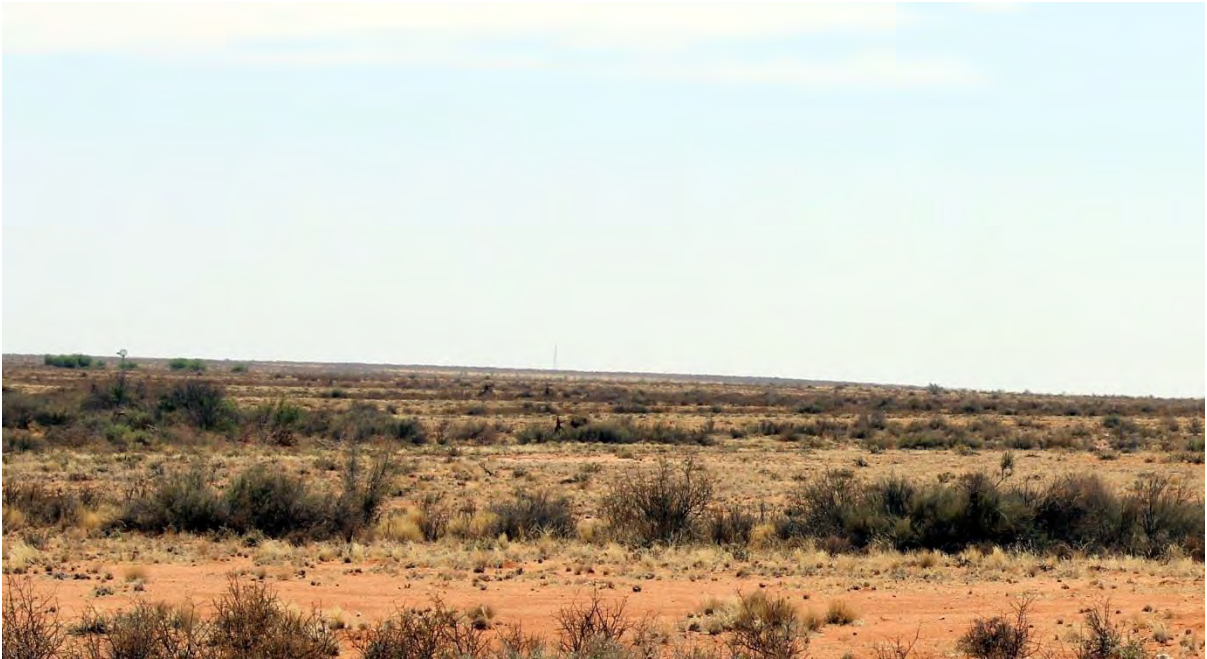
Figure 8.12: The tower at the Rugseer Siding as seen from photo site SCA011.
