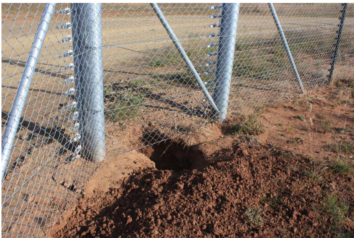
Figure 7.12: Fossorial movement under fences by larger animals, porcupines and Aardvark ( Orycteropus afer ).
