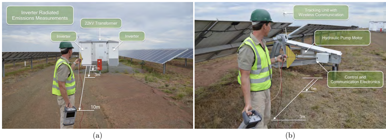
Figure 15: Radiated measurements of (a) Inverter and Transformer units and (b) Tracking Cabinet.
