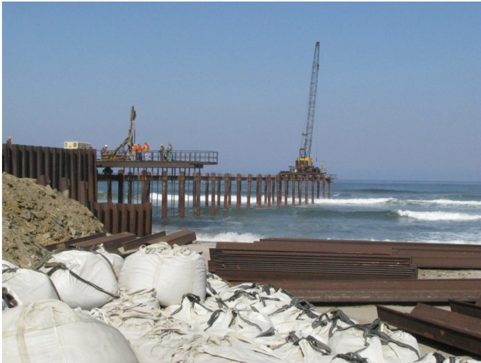
Figure 10-1 Example of a construction jetty for marine intake and outfall pipelines.
