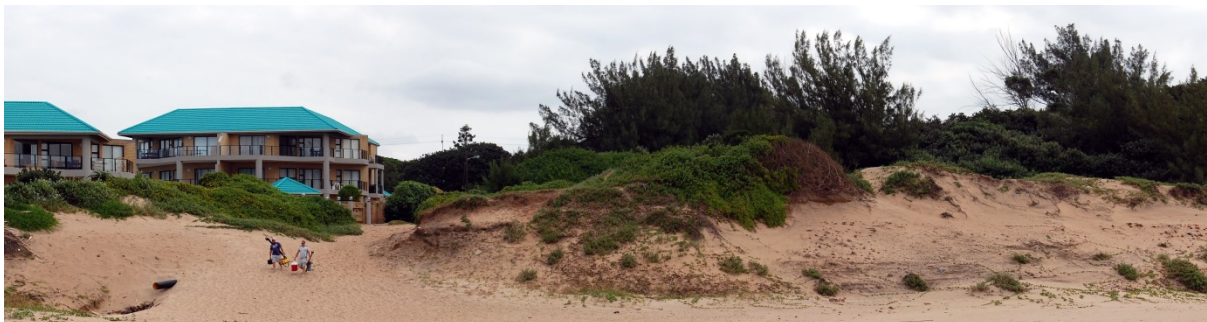
Figure 10-45 View from the beach at LVP014 near the proposed Jetty site. The Boardwalk residential complex is to the left and the proposed Pumpstation site to the right behind the dune.
