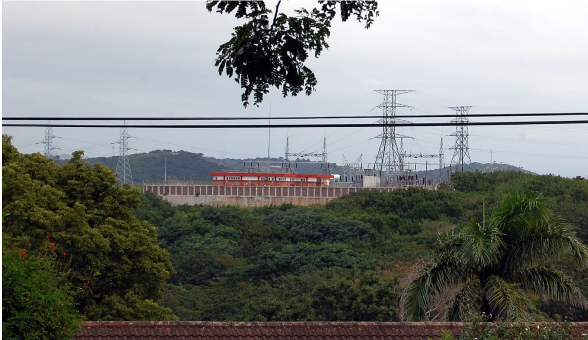
Figure 10-44 Kingsburgh Major Substation as seen from LVP012 in Astra Park.
