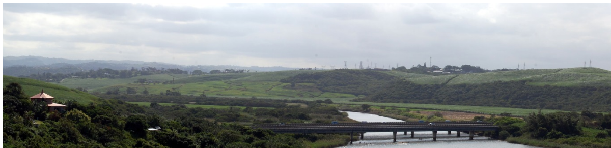
Figure 10-48 View north-west from LVP017, northern Illovo Beach, across the Lovu River floodplain. The Kingsburgh Major Substation is visible on the hills in the middle, as are the N2 and R102 bridges across the river.
