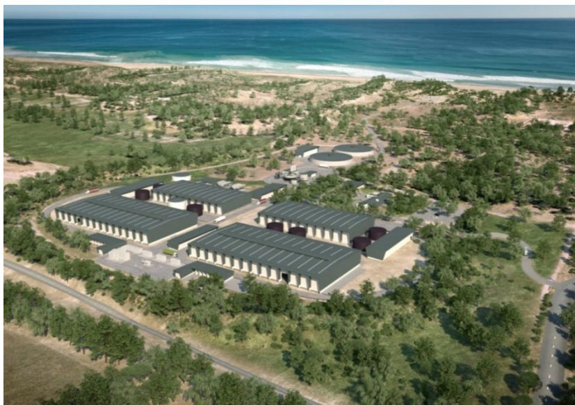
Figure 10-55 Another example of using a buffer of vegetation around a desalination plant. All industrial type structures are screened from public views.
