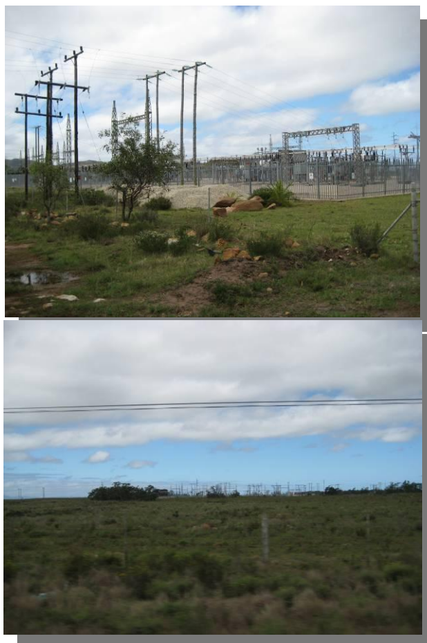
Figure 3.1: Melkhoutbosch substation, near the N2-R330 interchange north of Humansdorp
