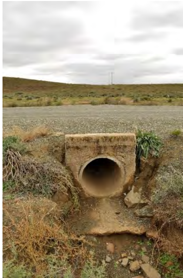
Plate 2: A view of an existing pipe culvert crossing on the R356 (32.7817023S 20.3044875E)
