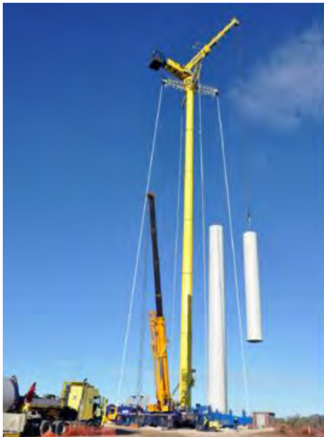
Figure 7: Cranes at work
