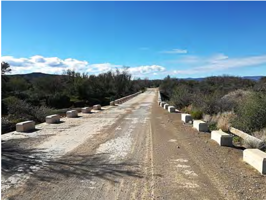
Figure 13: Narrow bridge on DR02249
