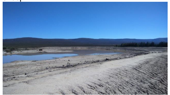
Plate 4: Earth-wall dam with water
