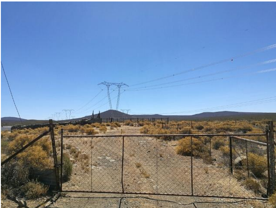
Figure 20: Power pylons near the R354
