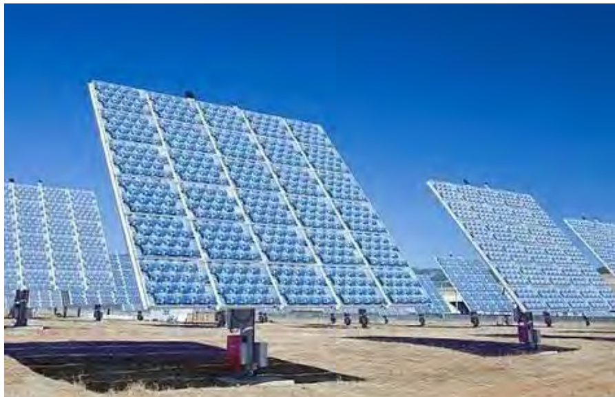
Figure 3.11: CPV energy facilities in the southern area of Spain 21
