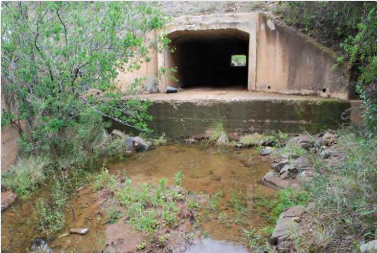
Plate 3: An example of an elevated culvert that has raised the level of the riverbed resulting in a form of habitat fragmentation.
