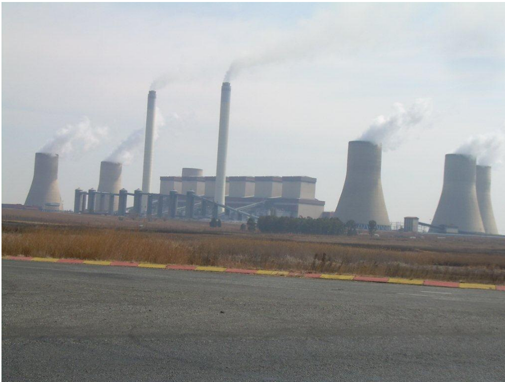
Figure 10.3: Tutuka Power Station forms the centre point of the study area, as the source of ash
