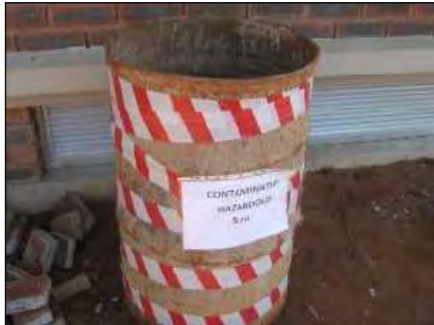
Figure 10: Example of 220ltr metal drum used to store contaminated soil.
