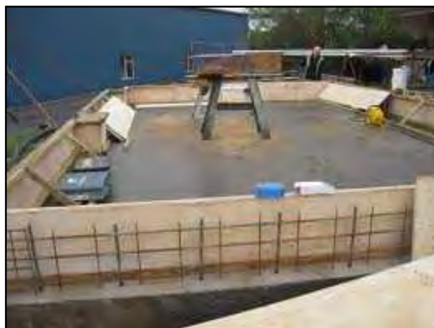
Figure 3: An example of a bunded area that should be used to contain the hazardous store area within the construction camp (source: www.oasis-environment.co.uk ).
