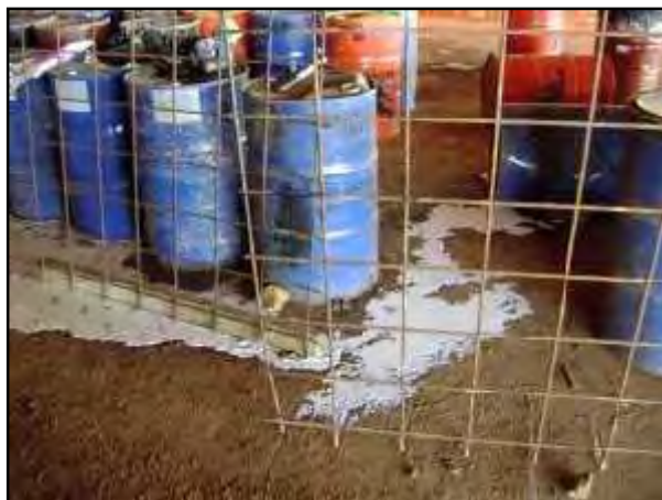
Figure 11: An example of hazardous material which has not been properly stored and is leaking on to bare soil. Hazardous material must always be kept separate from other storage areas and must be bunded.
