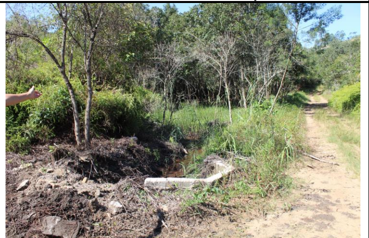
Figure 18: Weir Site 1: The drainage line flows under the existing road.
