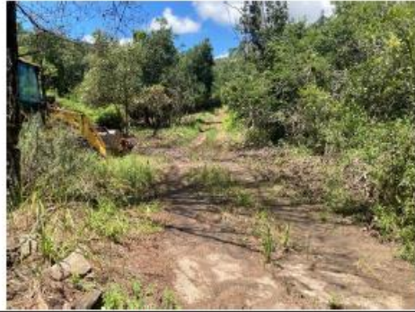
Photo 2: Weir 2 Site. See Bedrock on Surface
