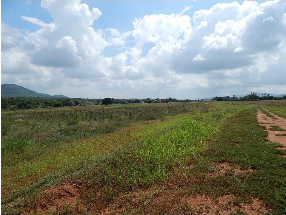
Fig. 11: The middle section, with the earth canal visible next to the road.
