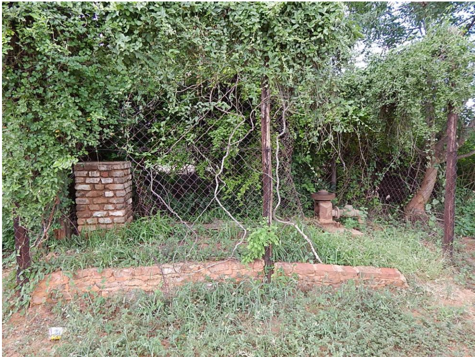
Fig. 20: The infrastructure of a water pump.
