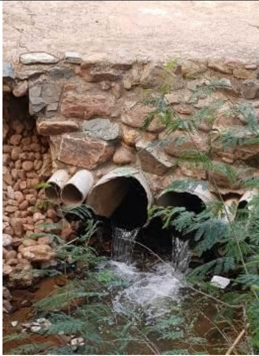
Plate 1: Existing bridge (barrier)
