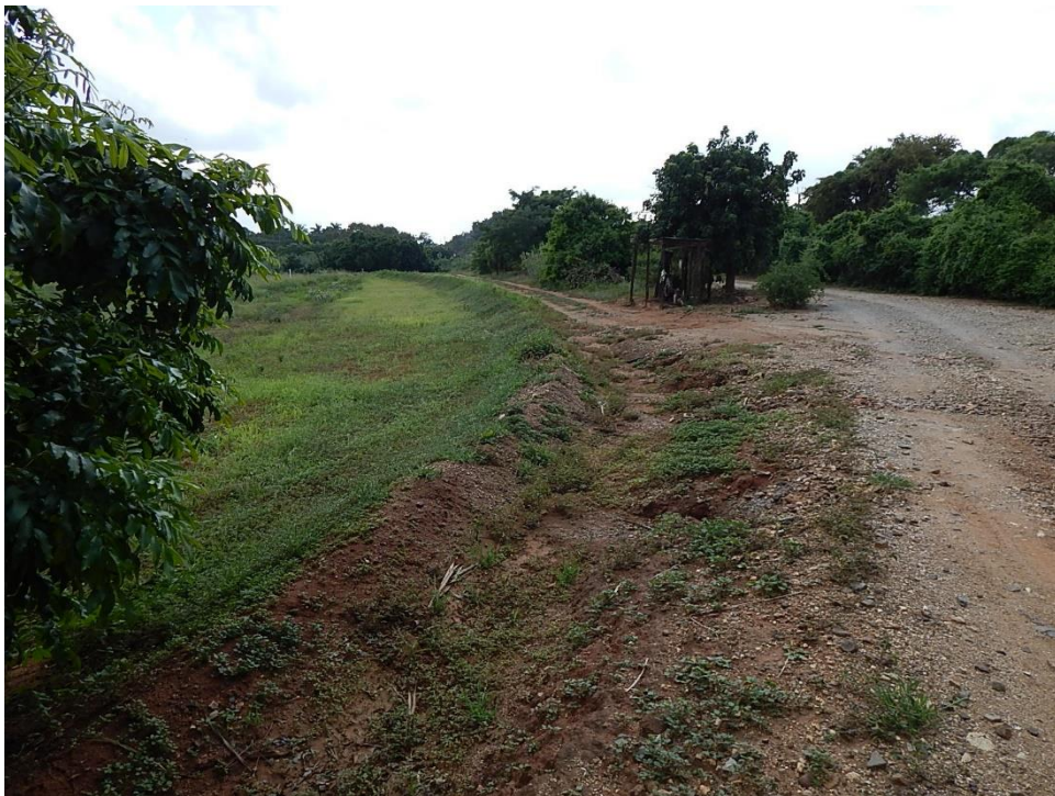
Fig. 22: The earth canal in the eastern section is visible next to the gravel road, facing east.
