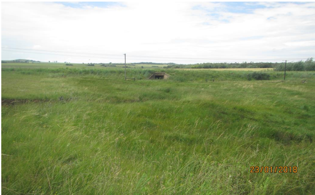
Photograph 10: View downstream of the dam wall after construction
