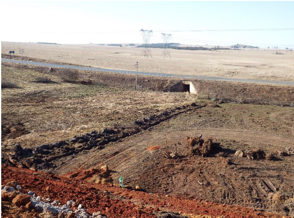
Photograph 9: View downstream of the dam wall during construction.
