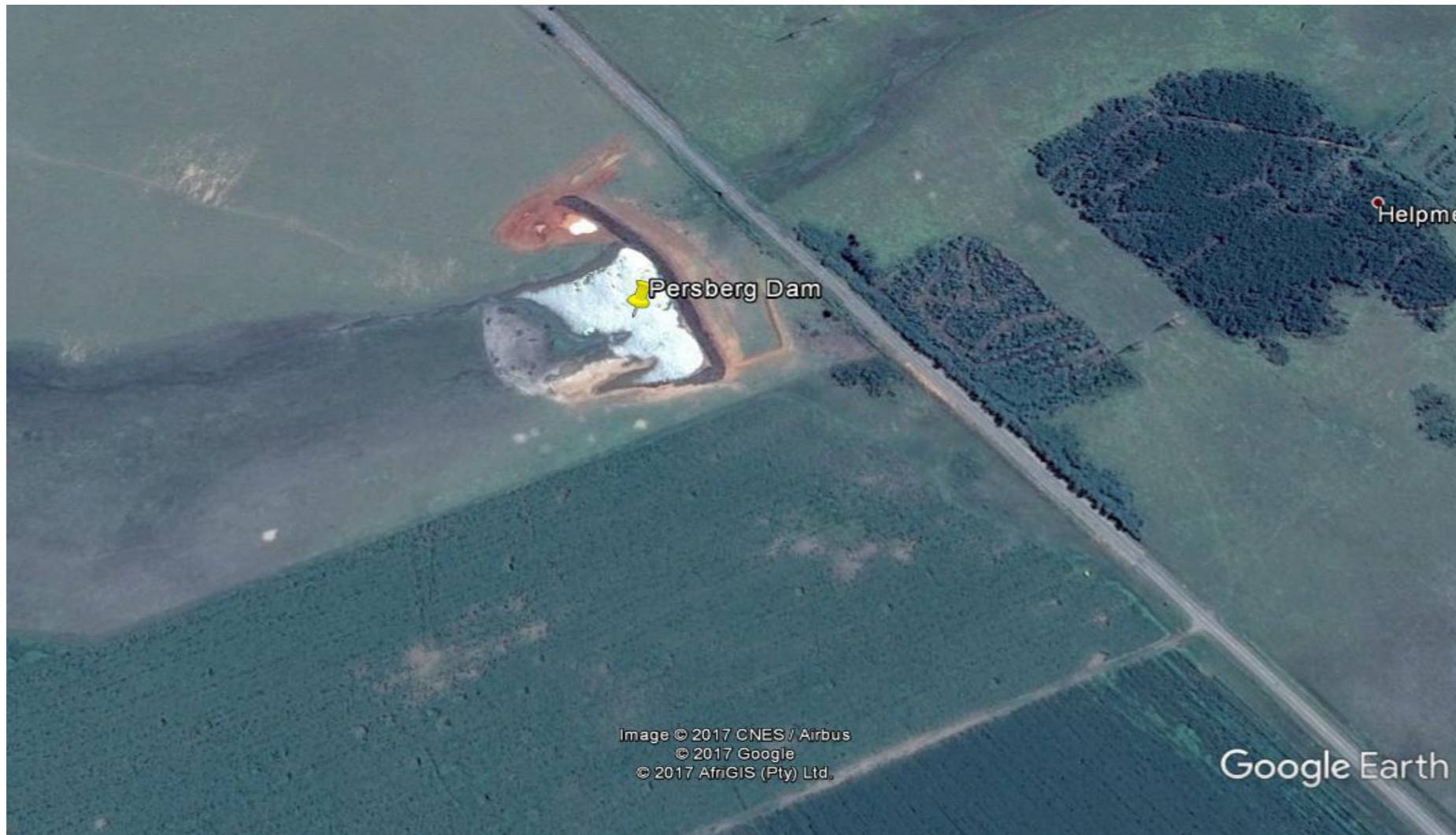
Figure 2: Aerial view of the Persberg dam site (courtesy Google Earth).
