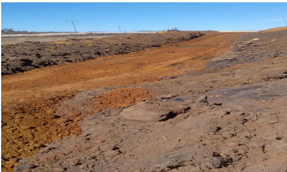
Photograph 6: Dam cut of key.
