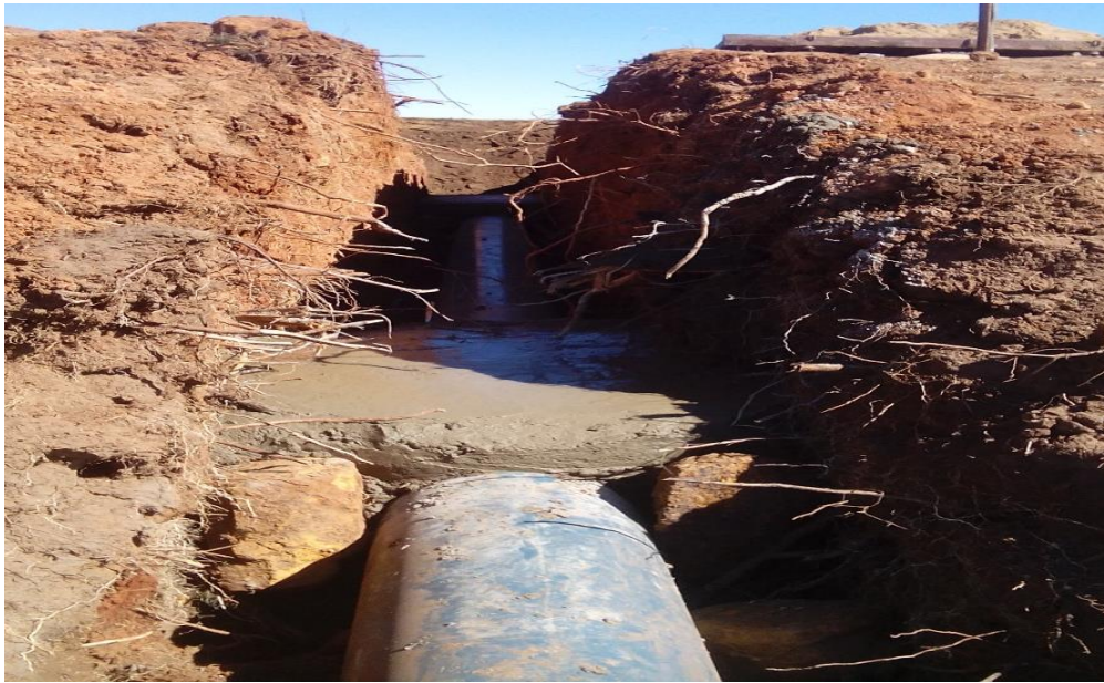
Photograph 7: Outlet pipe during construction of the dam wall.
