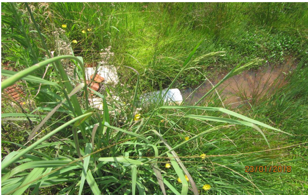
Photograph 8: Outlet pipe after construction of the dam wall.
