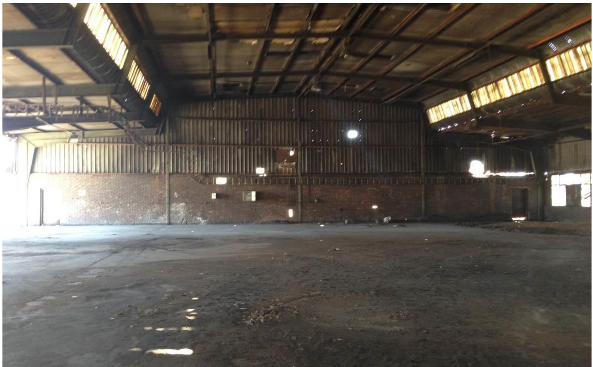
Figure 9: Inside of building 2
