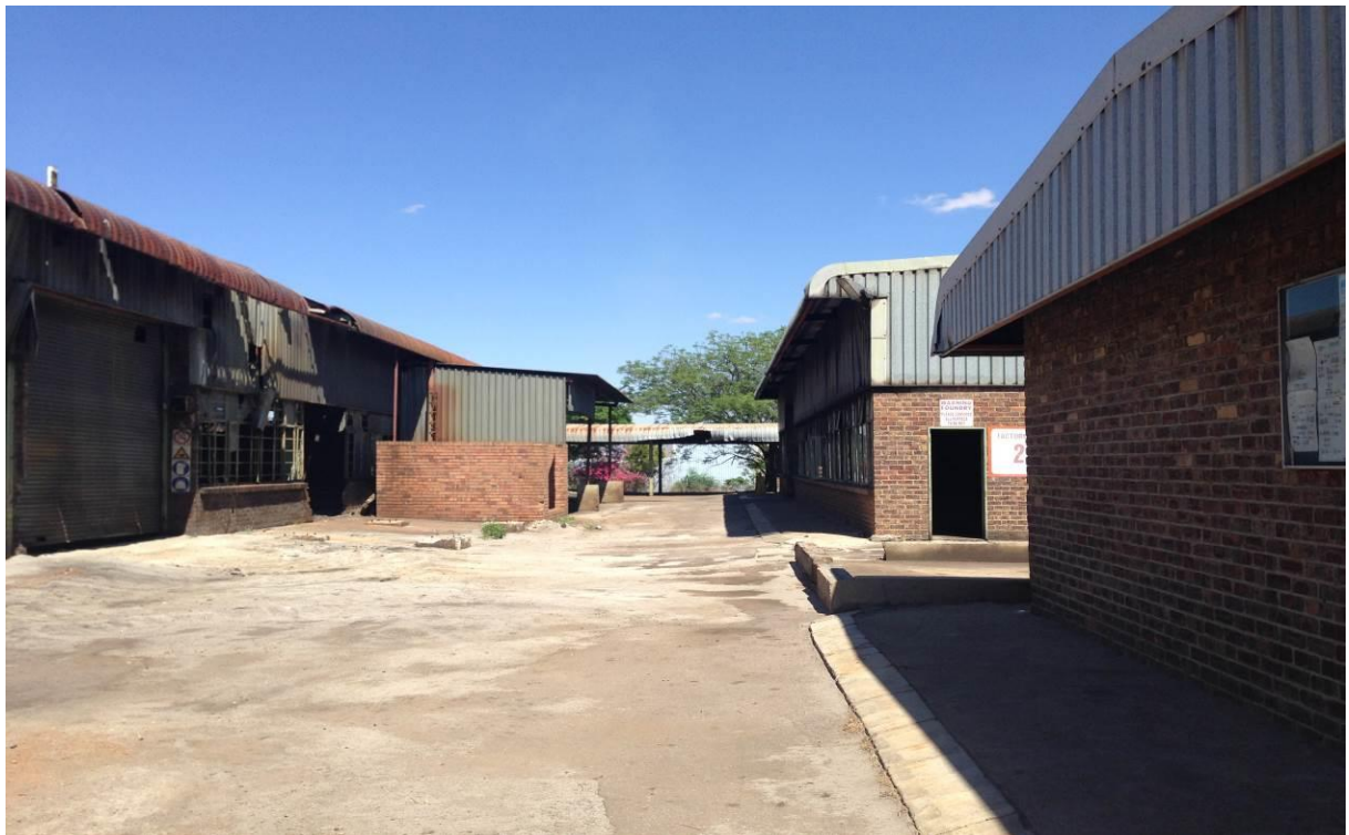
Figure 7: Existing buildings (building 3 at the back on the right of the photograph)
