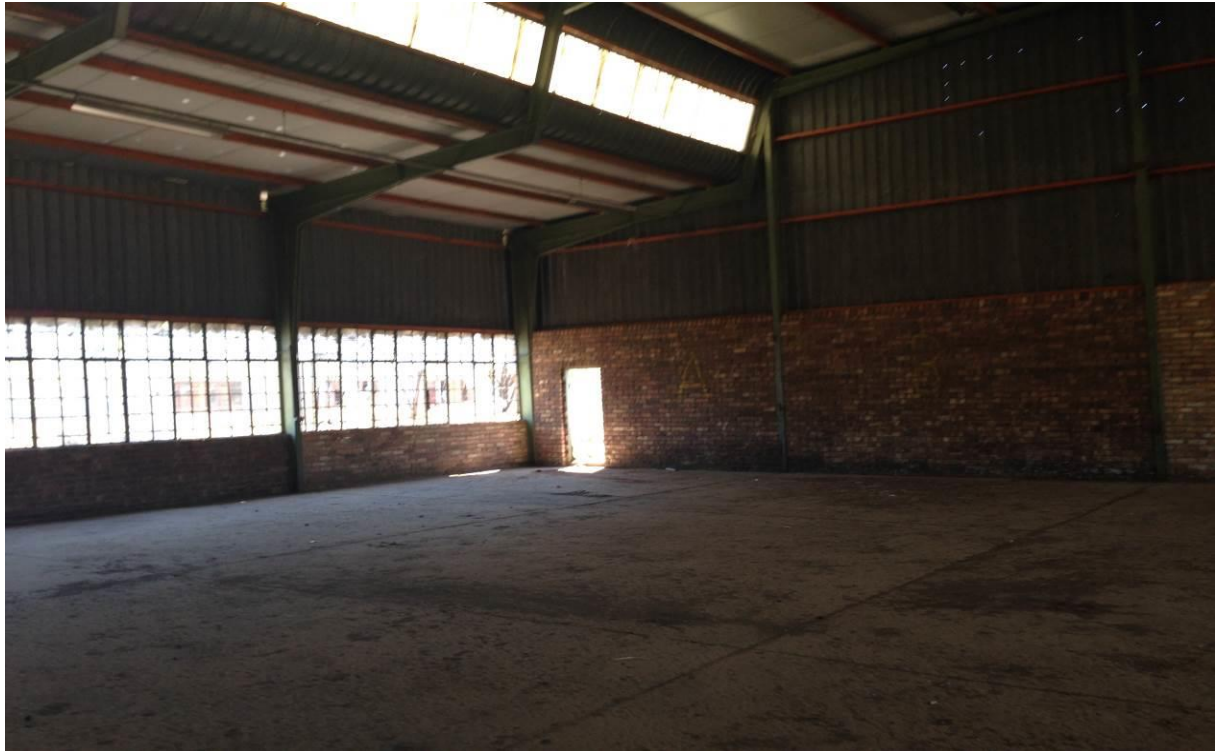
Figure 8: Inside of building 1
