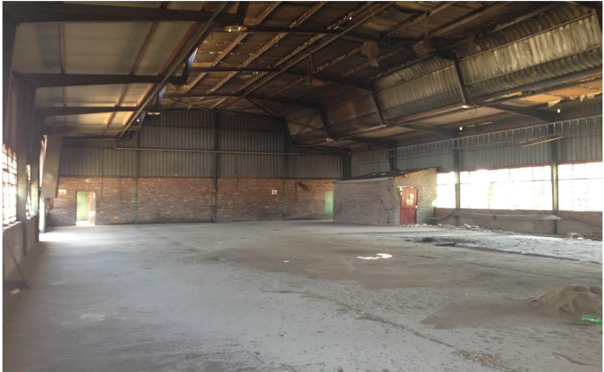
Figure 10: Inside of building 3
