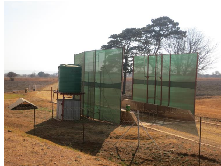
b – Typical disinfection spray station for incoming vehicles
