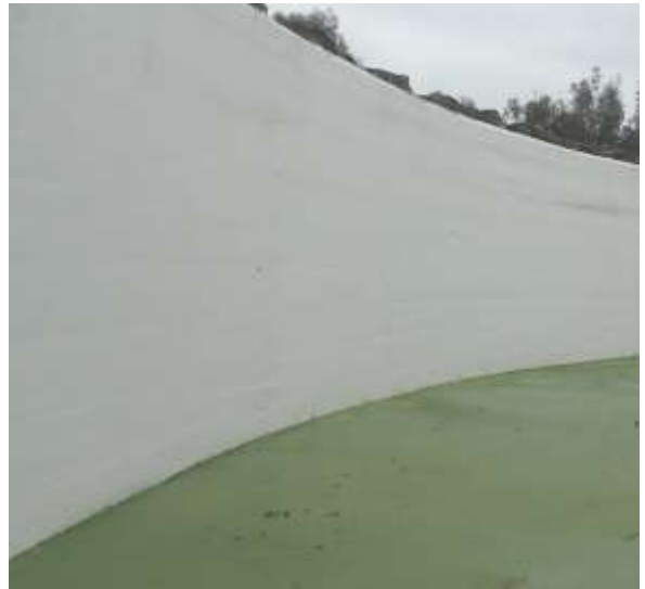
Fig 5; The plat form with no drainage
