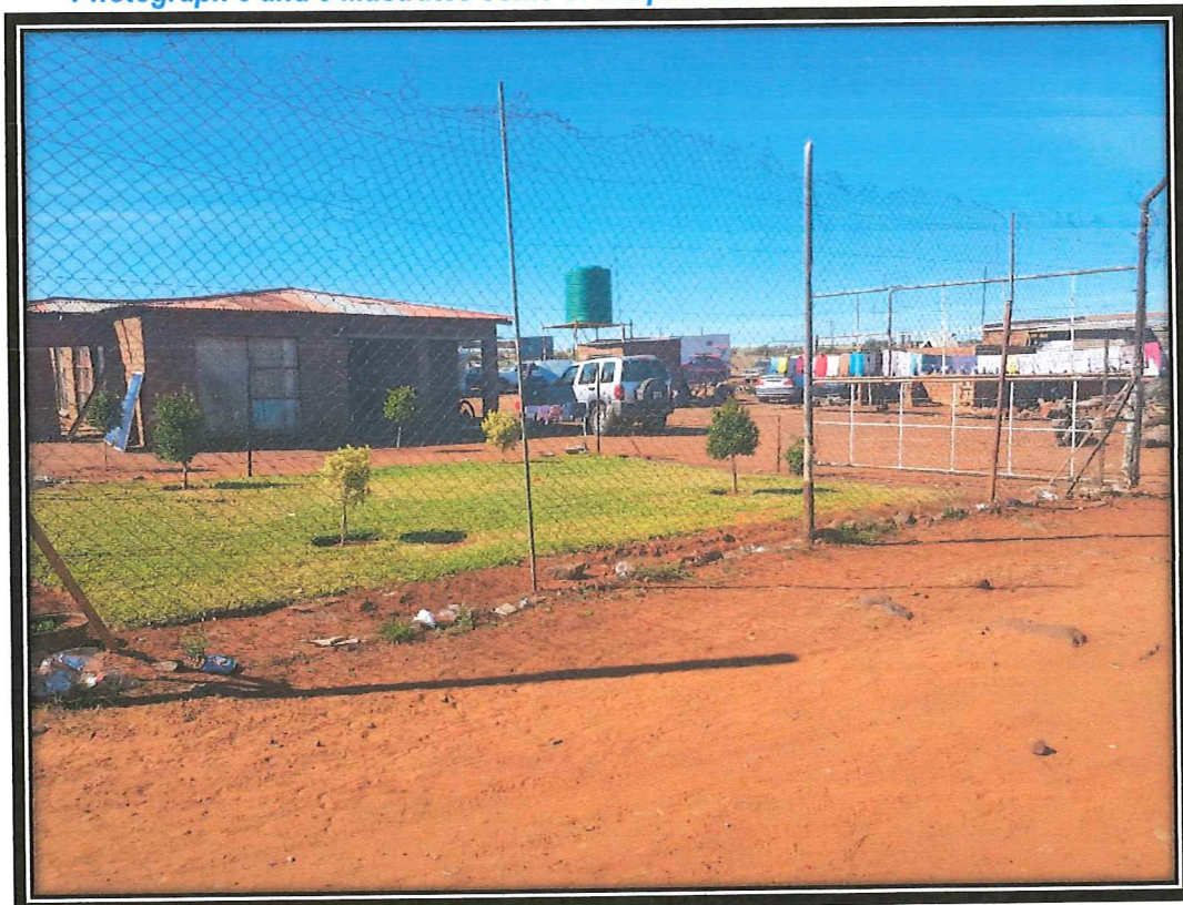
Photograph 8 and 9 illustrates some of the permanent structures found on site
