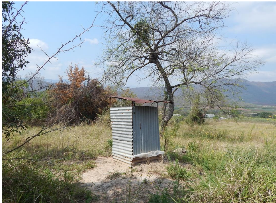
Fig. 12: A pit toilet is still visible near the hostel, and close to the southern border.
