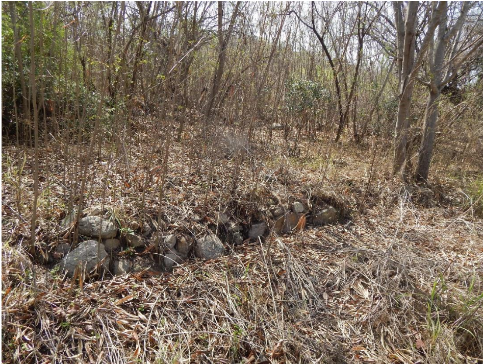
Fig. 11: Stone foundations towards the east, indicate where more compound/hostel houses were, before they were demolished. It is currently covered with alien vegetation.
