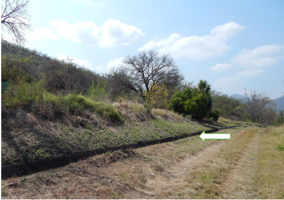
Fig. 7: A long concrete water canal forms the southern boundary of study area 1.
