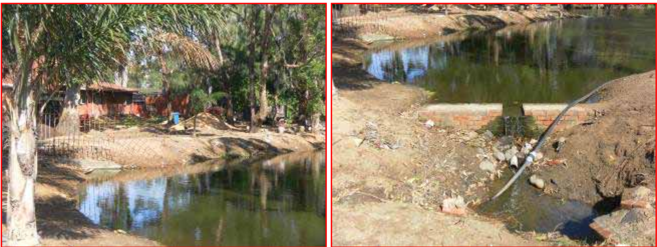
Figure 12: Photographs of the existing “duck pond” located in the south-west corner of the site where chrome remediation activities are being carried out.
