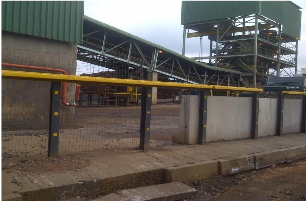
Figure 6: The conveyor system used at the facility
