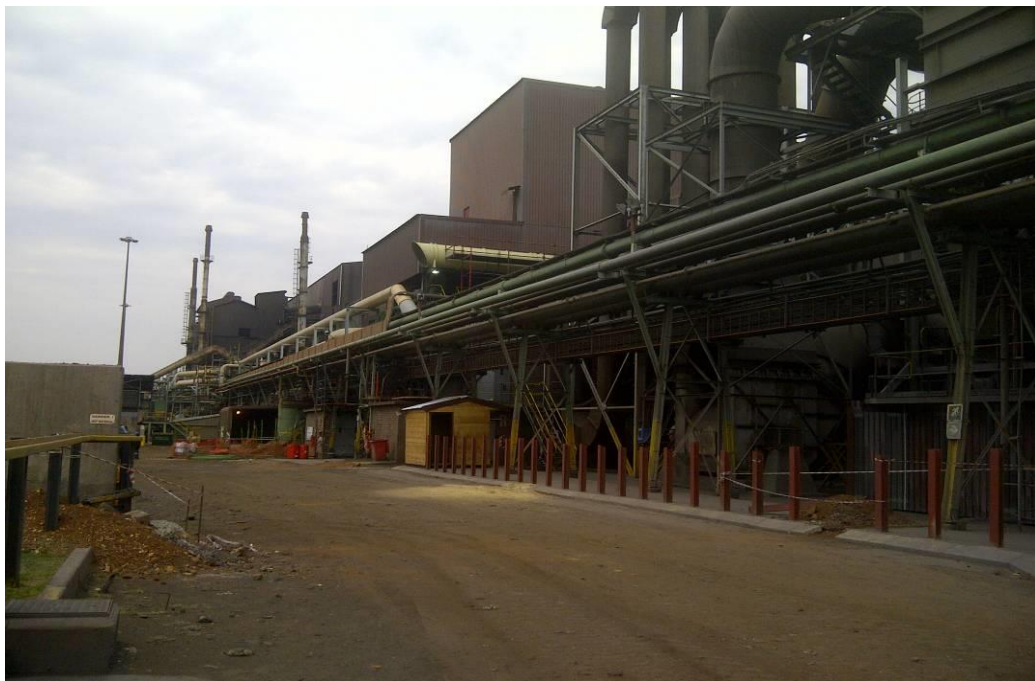
Figure 7: DMS Powders plant (1)
