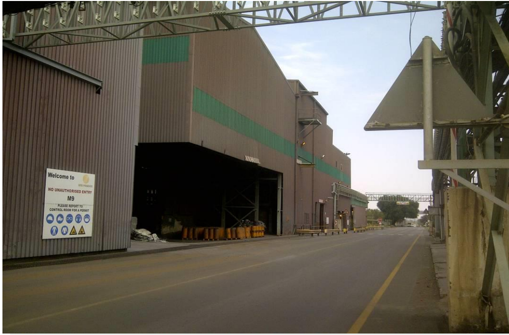
Figure 8: DMS Powders plant (2)
