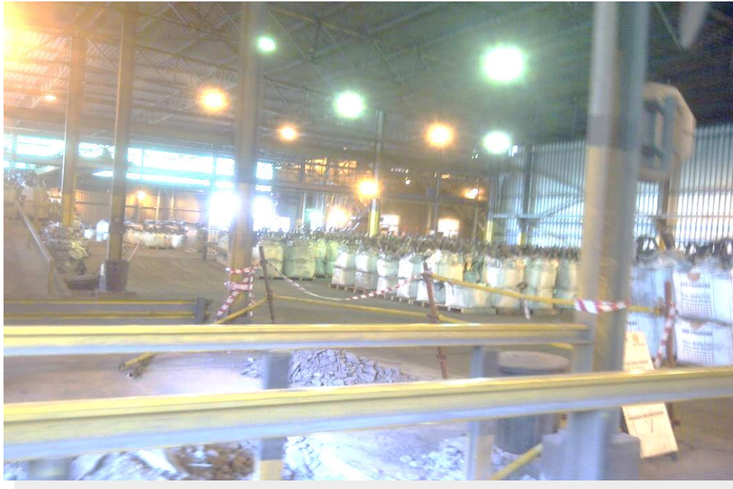
Figure 10: Product storage area
