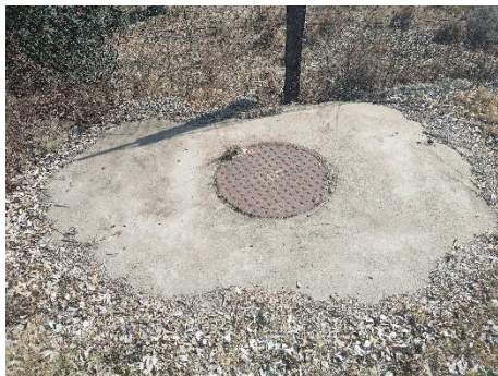
Figure 09: Manhole in Viljoen Street
