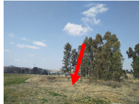
Figure 20: Small Dam (Retention)
