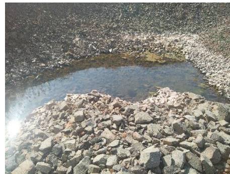
Figure 06: Water present at Quarry
