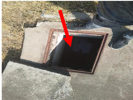
Figure 14: STW Drain in Springbok Ave.
