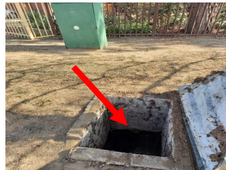
Figure 10: Closest Sewer Chamber
