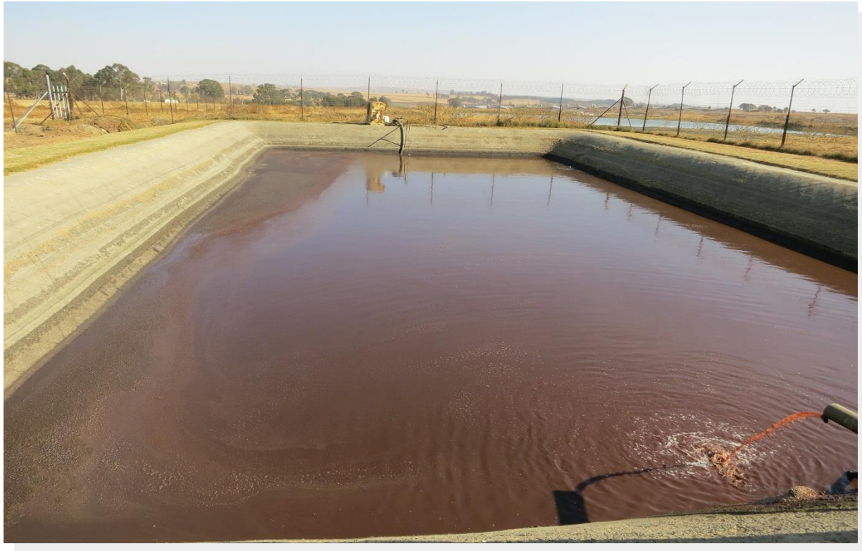
Figure 28: Wastewater overflowing from the anaerobic pond flows into this settling pond
