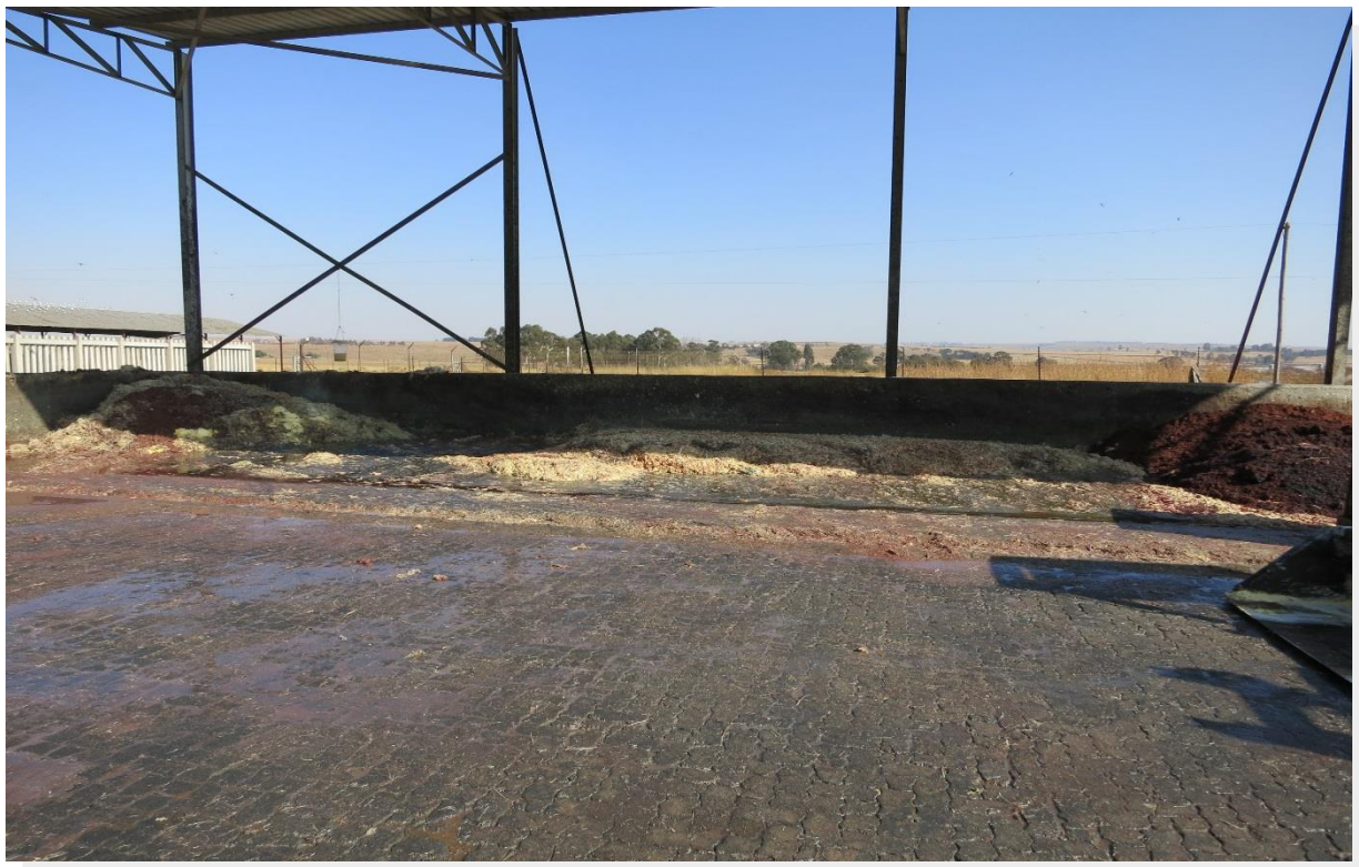
Figure 15: The current poultry waste storage area (bunker)
