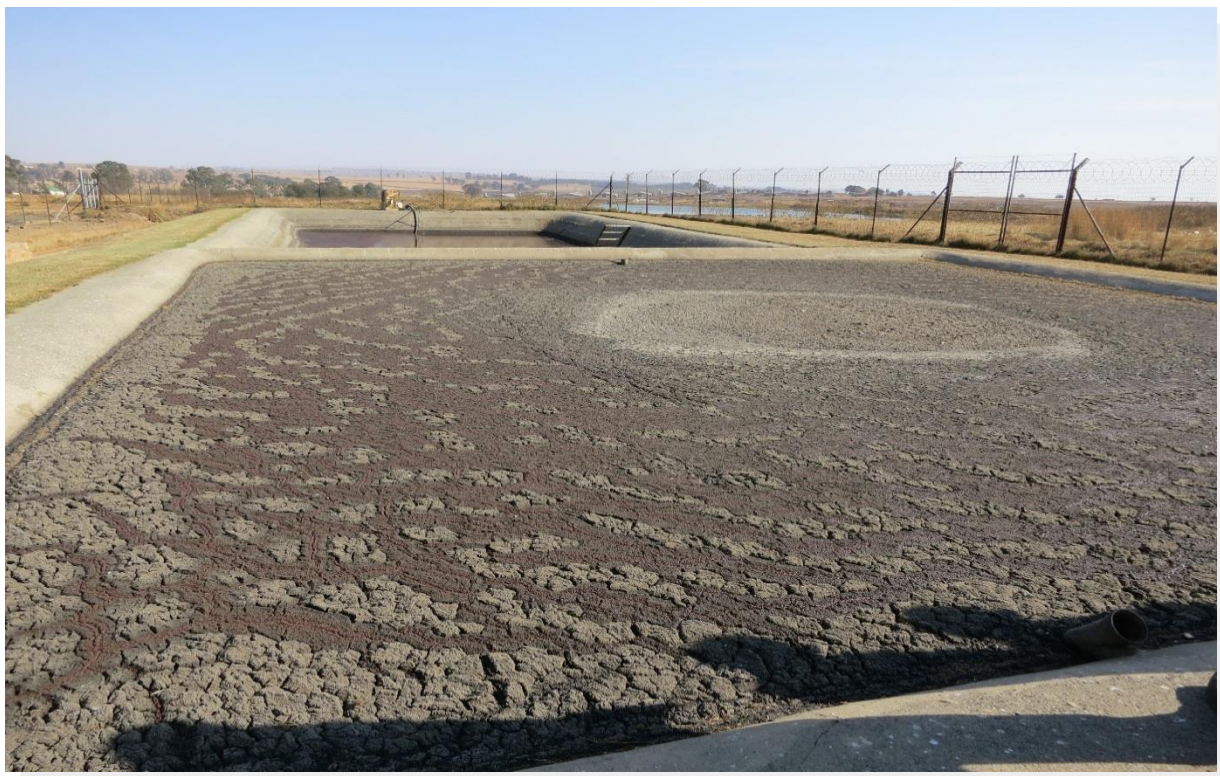
Figure 27: The anaerobic pond into which wastewater from the rendering facility flows
