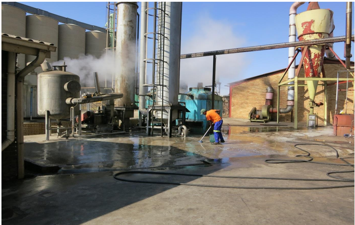
Figure 23: The current condensers
