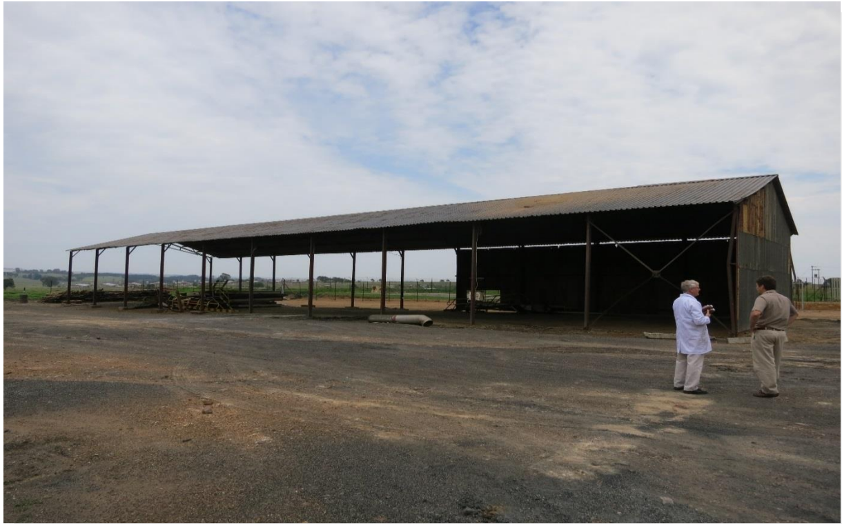
Figure 30: The first storage shed that will be removed to make room for the proposed second processing plant
