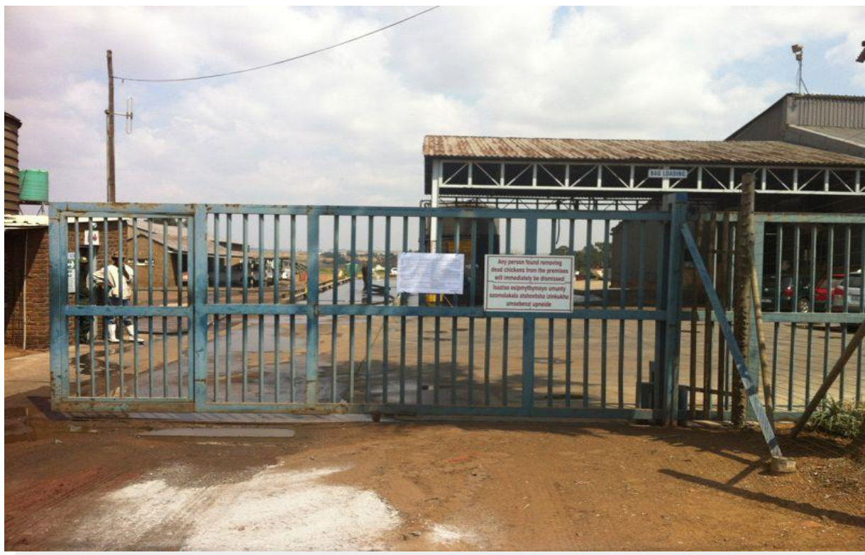
Figure 82: Site notice 1 at the entrance gate to the rendering facility
