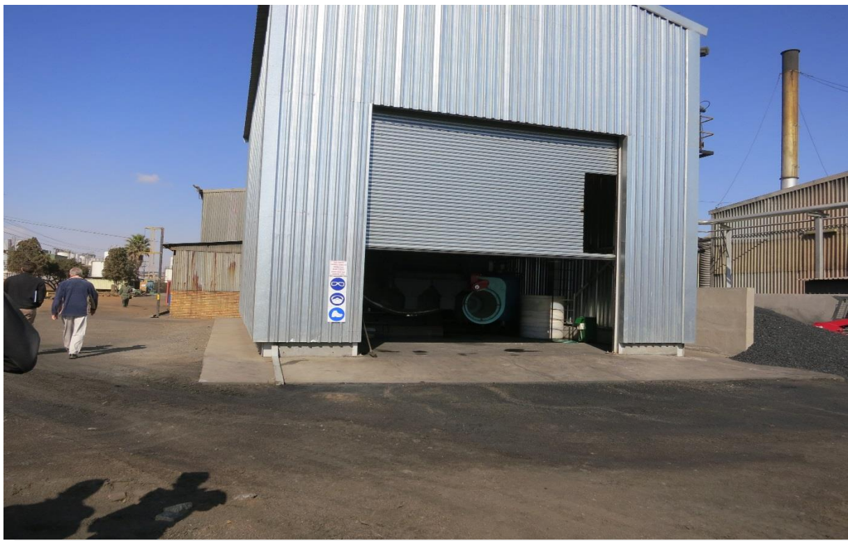
Figure 13: The 10 ton coal-fired boiler
