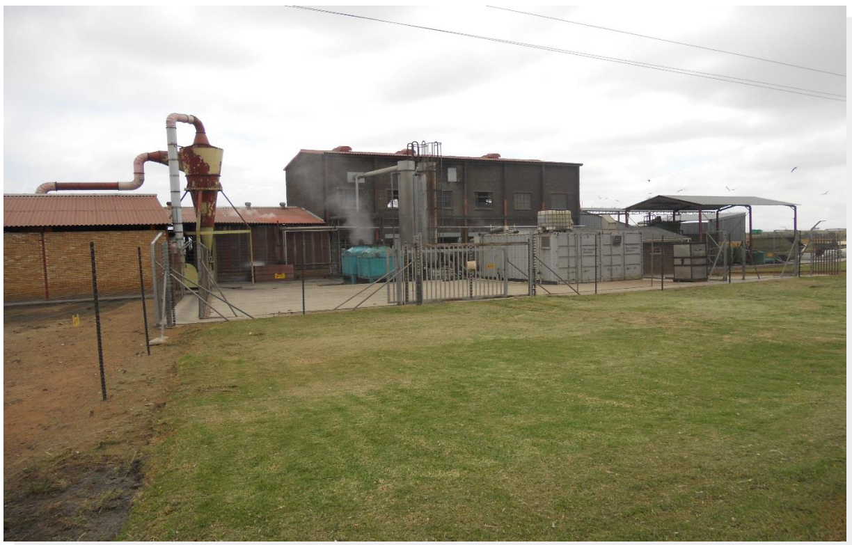
Figure 7: View of the current rendering facility from the east
