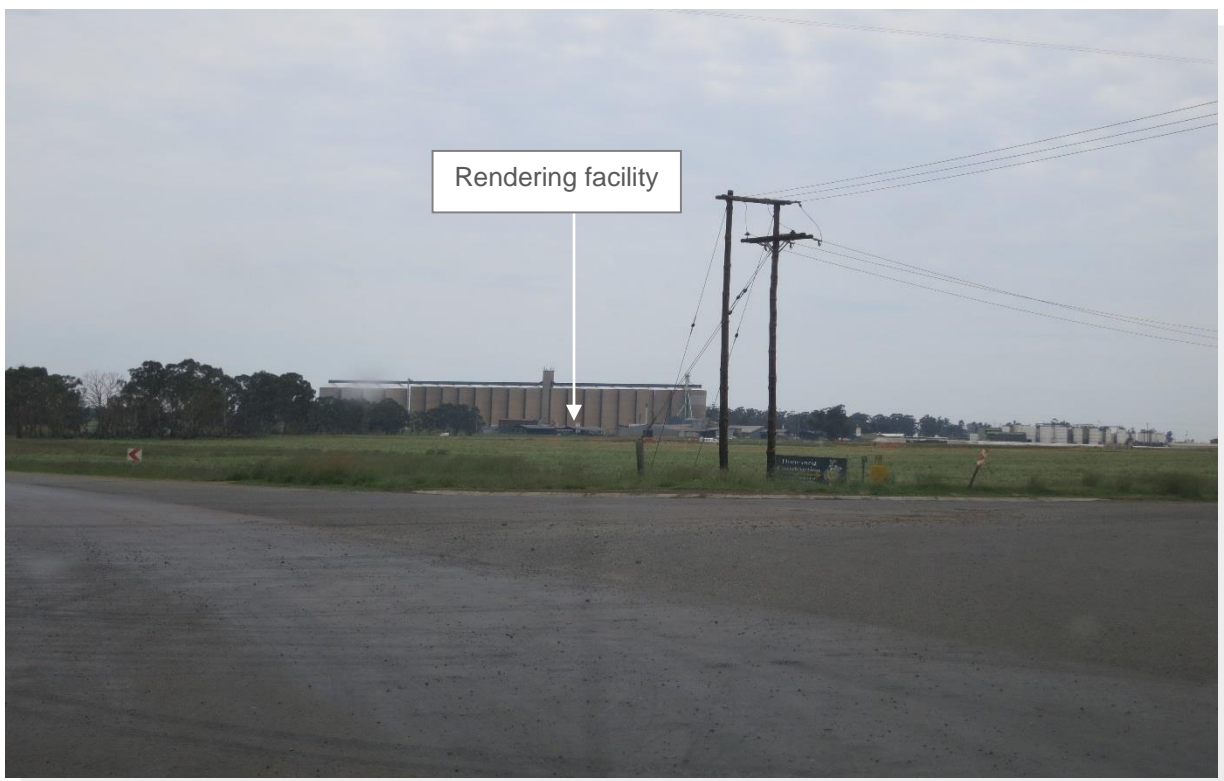
Figure 71: View of the rendering facility from the south-west.
