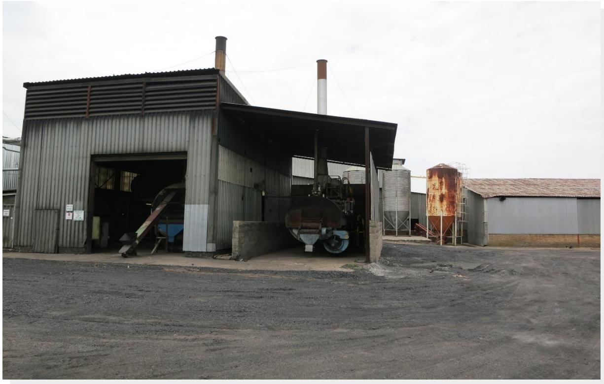
Figure 12: The 6 ton (left) and 3 ton (right) back-up coal-fired boilers
