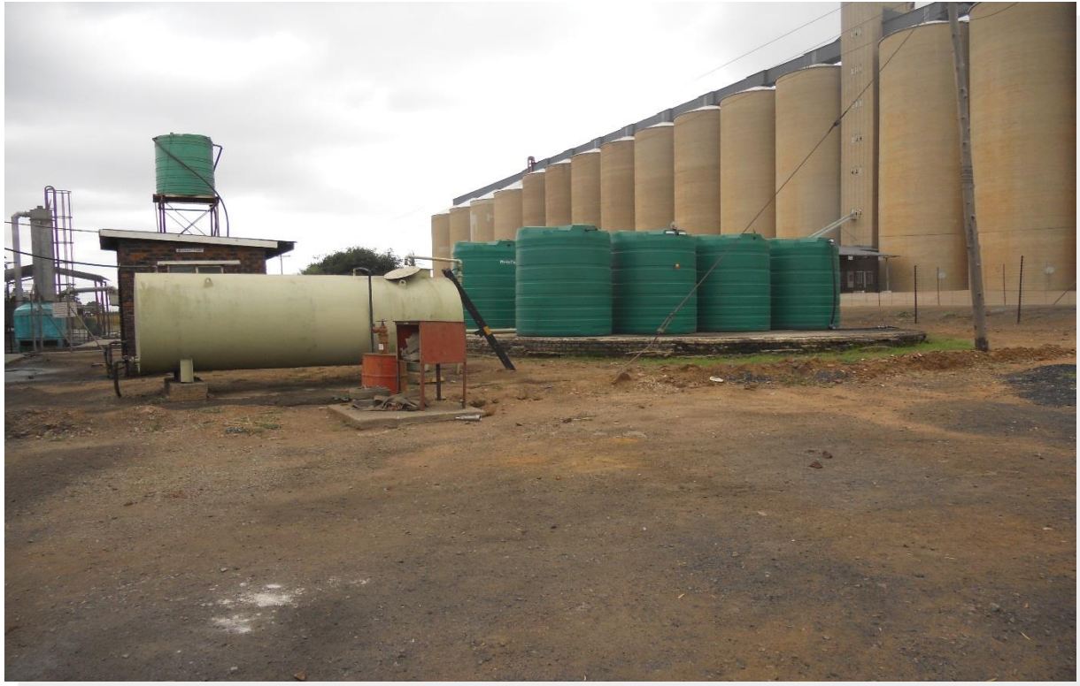
Figure 10: The JoJo tanks where water from the reservoir is stored
