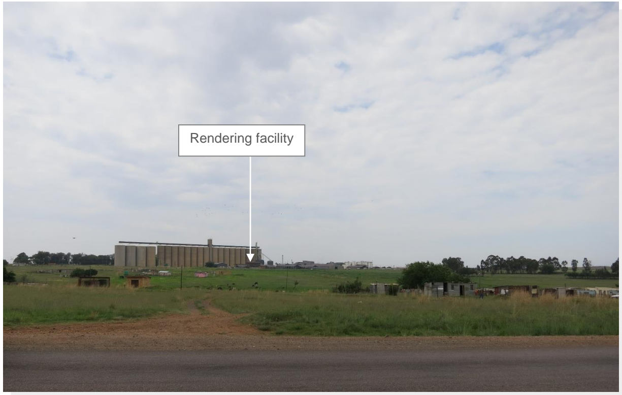
Figure 69: View of the rendering facility from the R555 (west of the facility)
