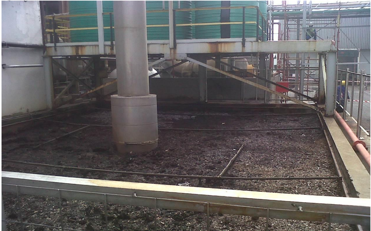
Figure 8: Bio-filter system outside the rendering plant
