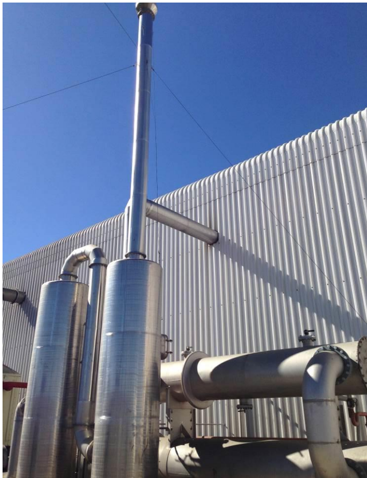
Figure 7: Ozone oxidation system on outside of rendering plant
