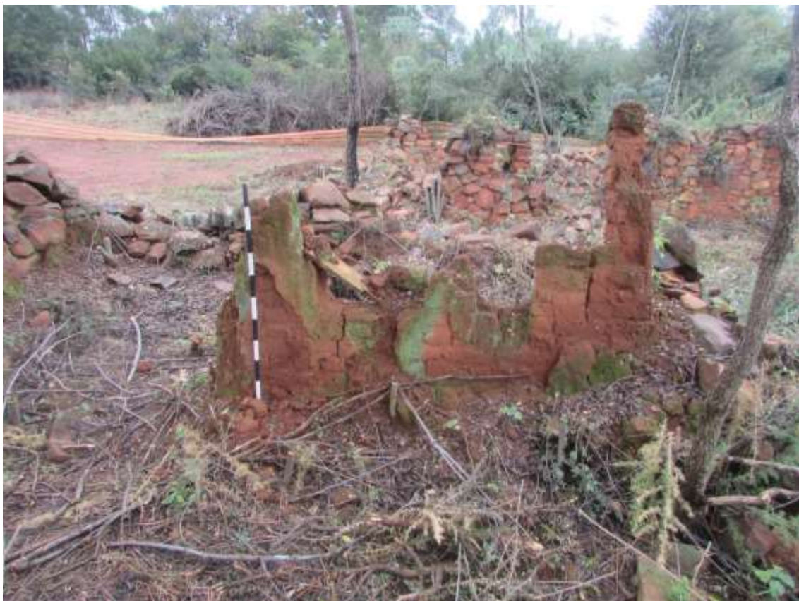
Figure 18: A view of one of the structures showing the combination of stone and clay brick walling used.
