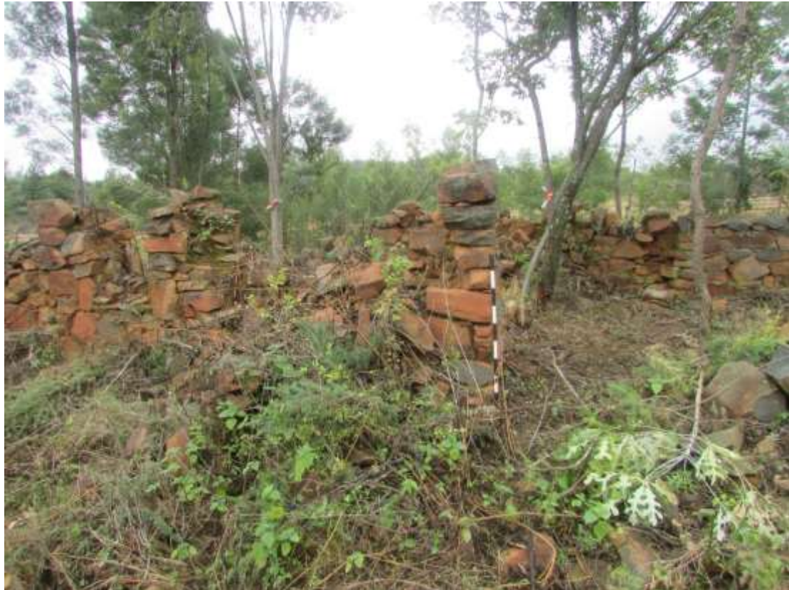
Figure 17: A view of one the 3-roomed structures/houses on the site.
