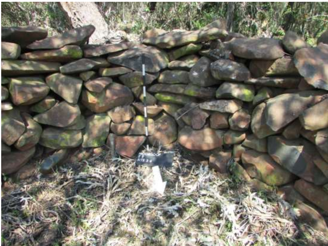
Figure 13: A section of well-preserved walling.
