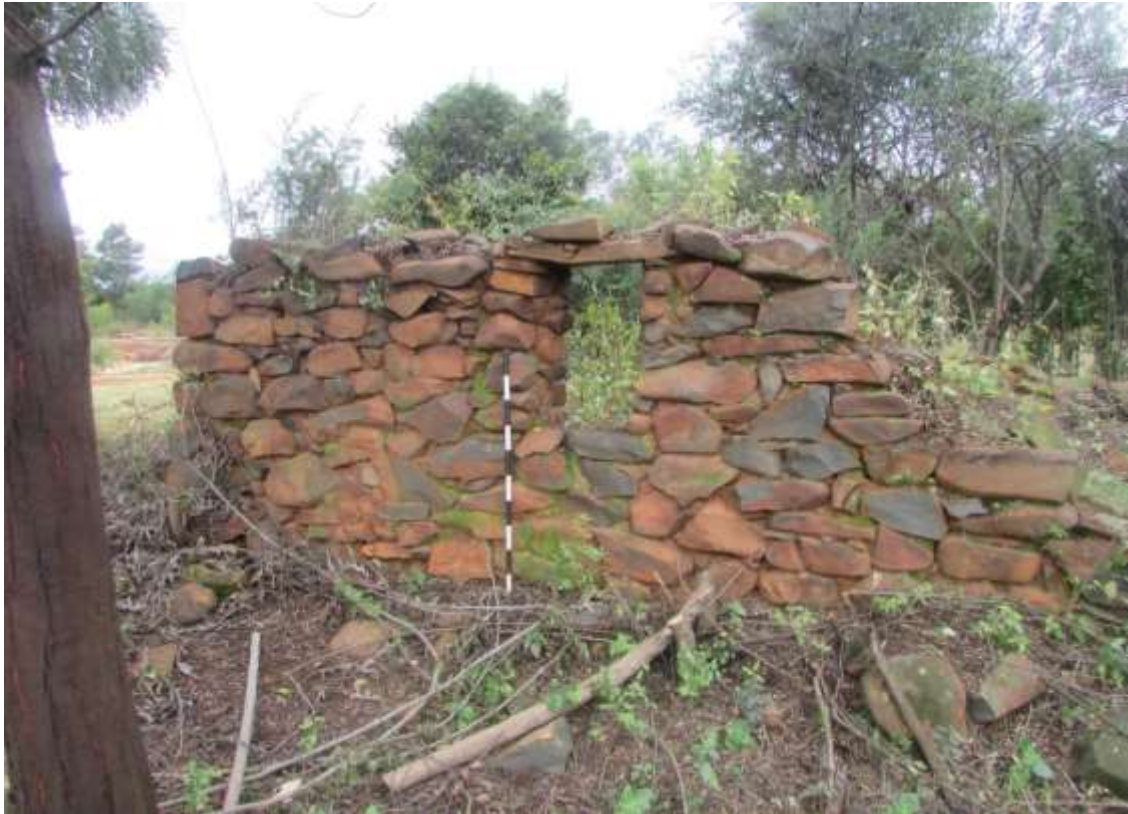
Figure 20: A window at one of the structures.
