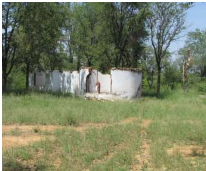
Fig.14: One of the abandoned structures on Site 20.
