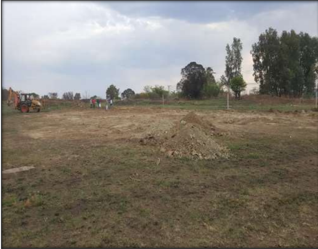
Fig.16: The main cemetery area after exhumation and removal has been completed.
