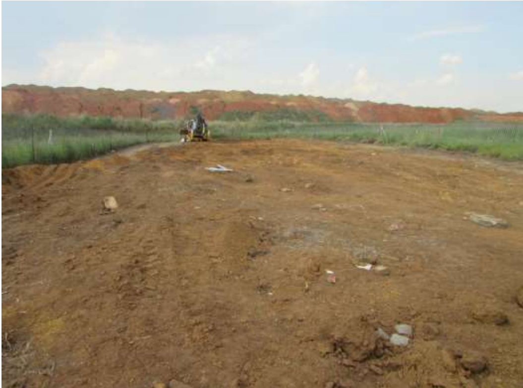
Figure 5: Site OI West after completion of the work.
