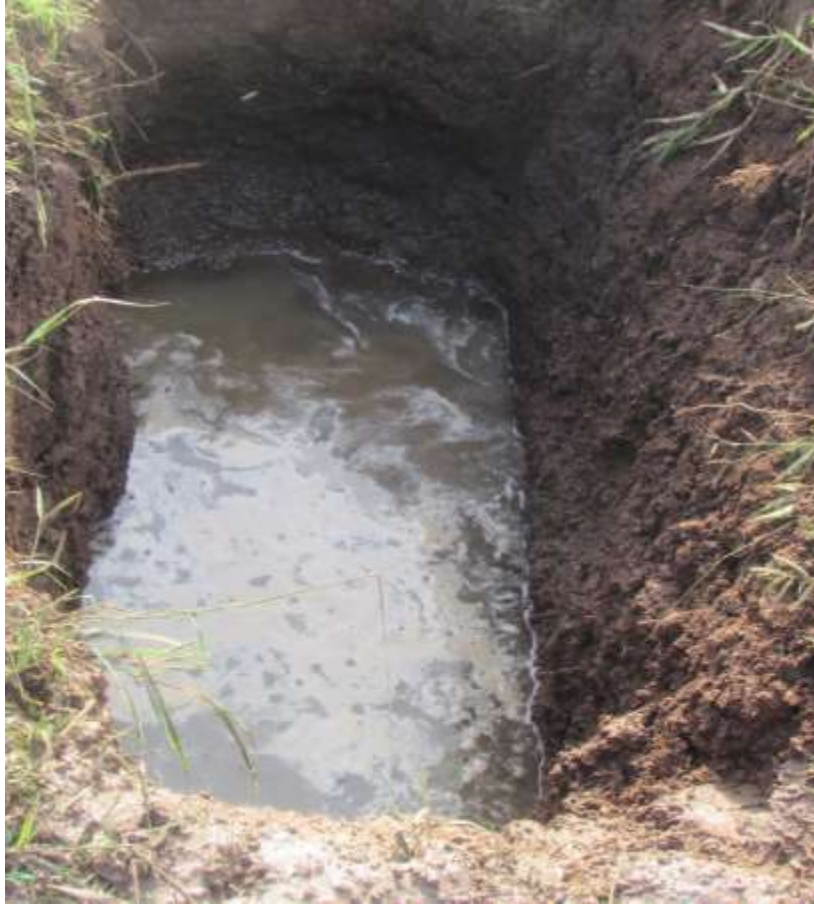
Figure 32: Once the exhumation commenced water constantly kept seeping in from the bottom.
