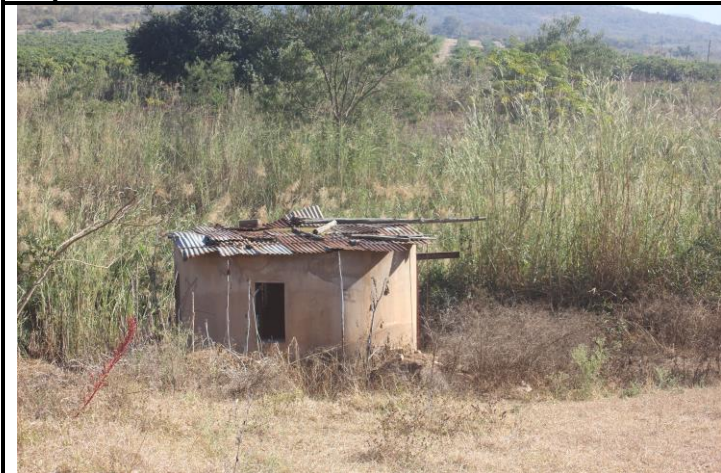
Figure 17: Old Pump Station: Kotze Property. Near preferred site.
