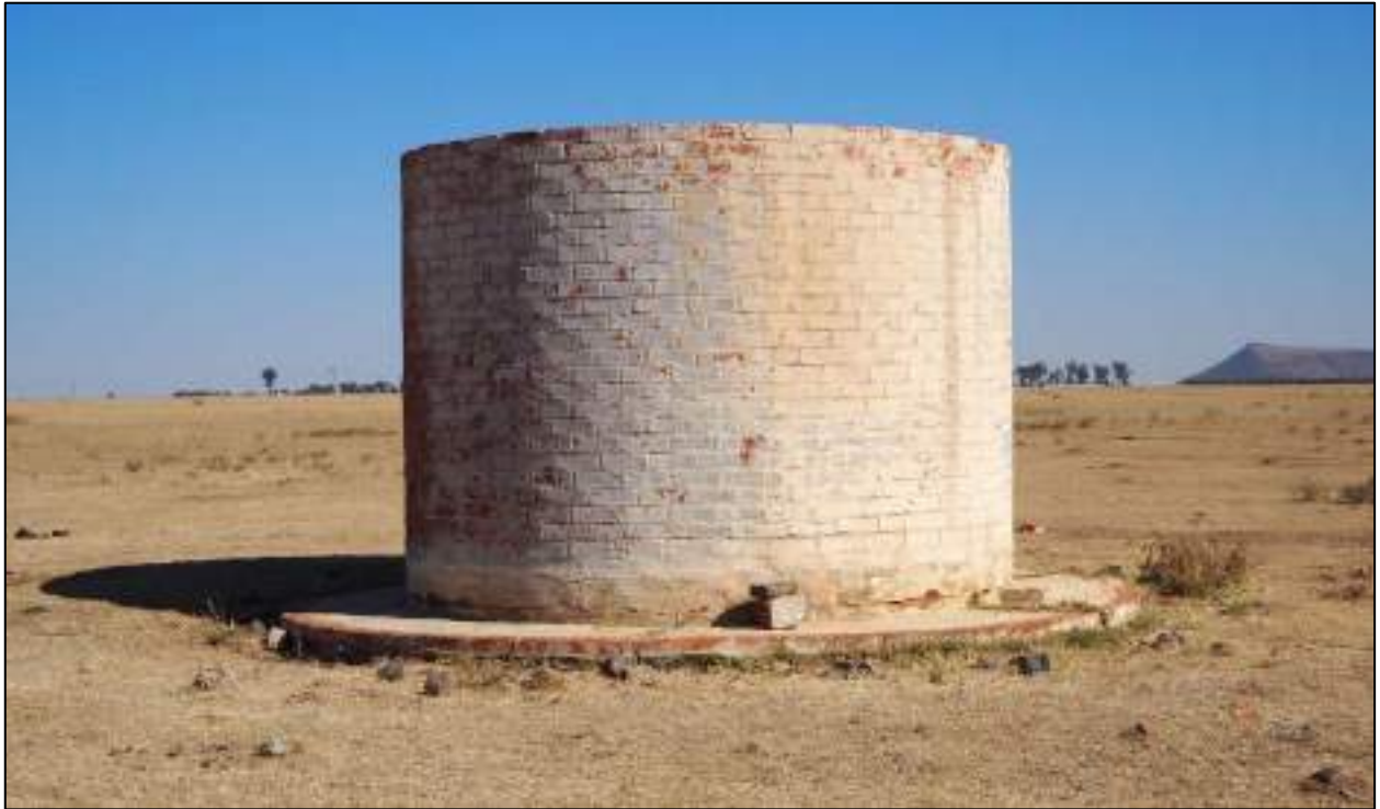
Figure 21. Water cistern close up
