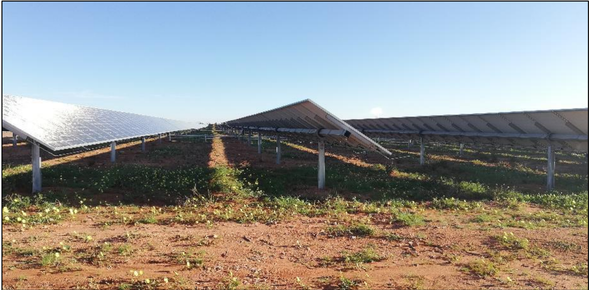
Figure 2: Photographic example of what the proposed PV could look like as fixed and single portrait model on a tracker.
