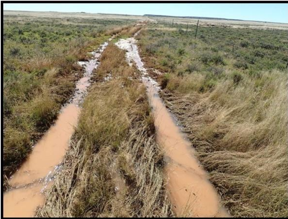
Figure 37: The clayey soils and most noticeably the Swartland and Valsrivier soils may restrict vehicle movement during the wet season.
