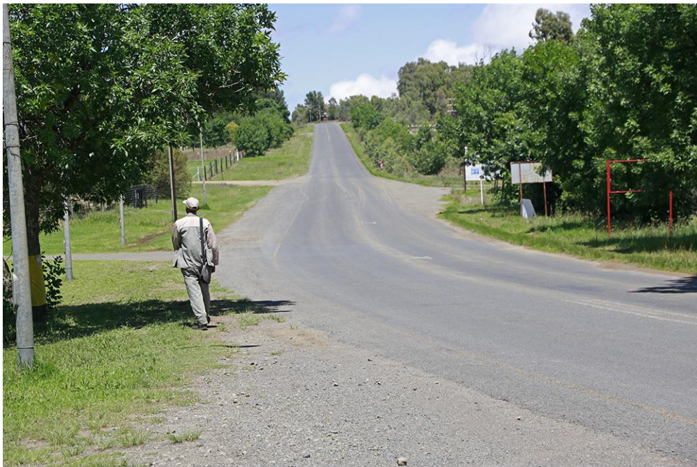
Photo 1: A116 as seen towards the south
