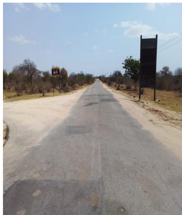
Photo 4: Road D4419 between Hluvukani and Nyeleti
