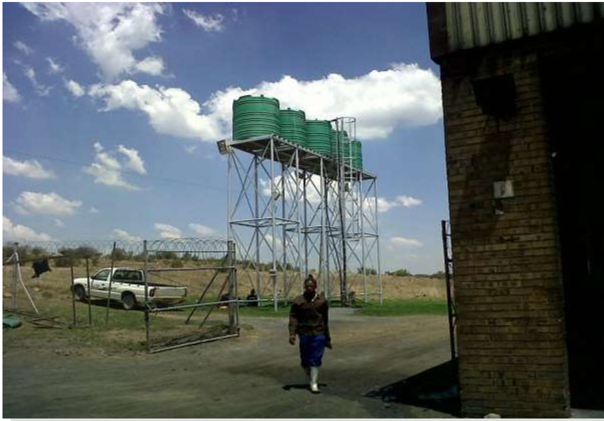
Figure 5: JoJo tanks used to store borehole water from an adjacent property
