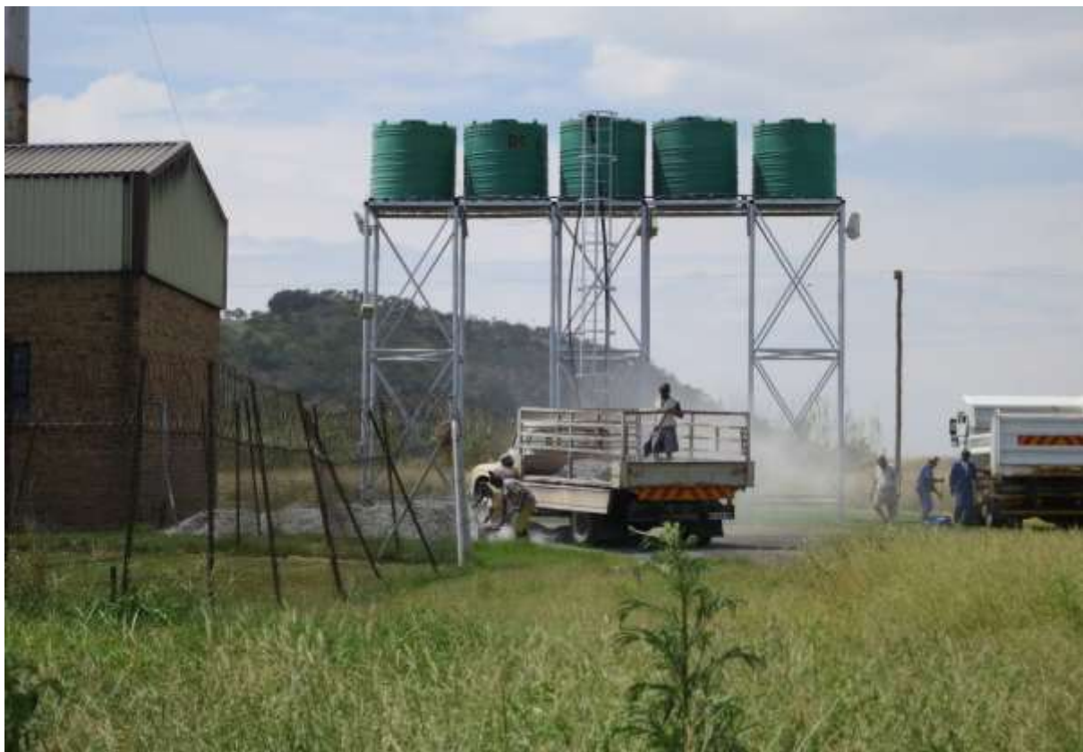
Figure 17: Removal of boiler ash
