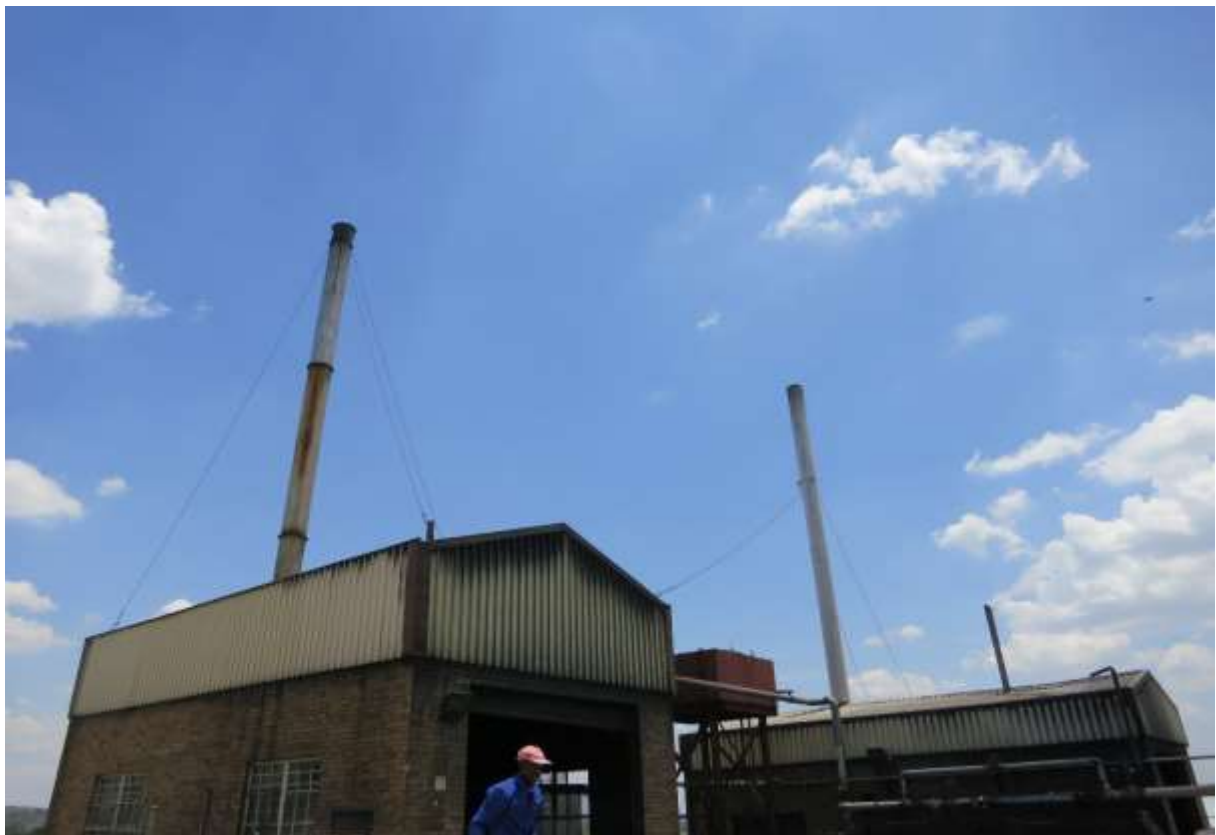
Figure 9: The two boiler stacks
