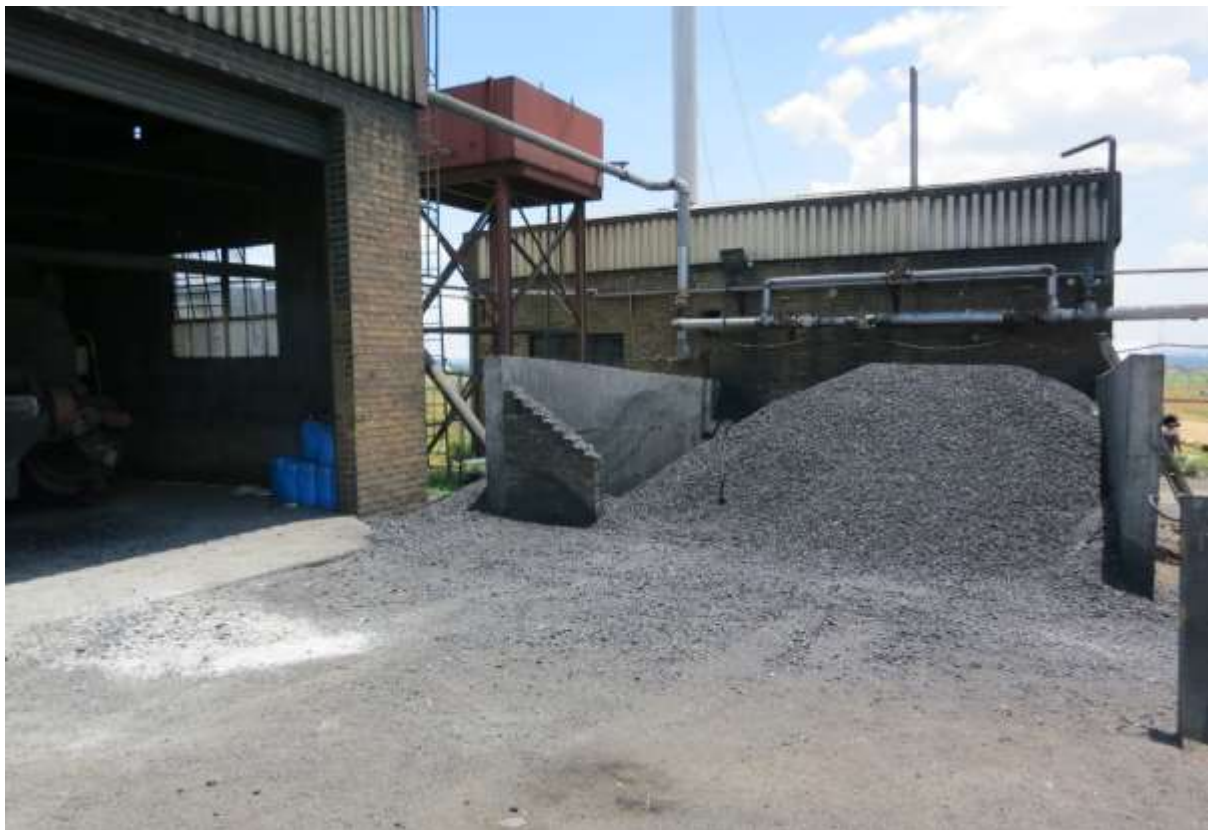
Figure 7: The coal storage bunker
