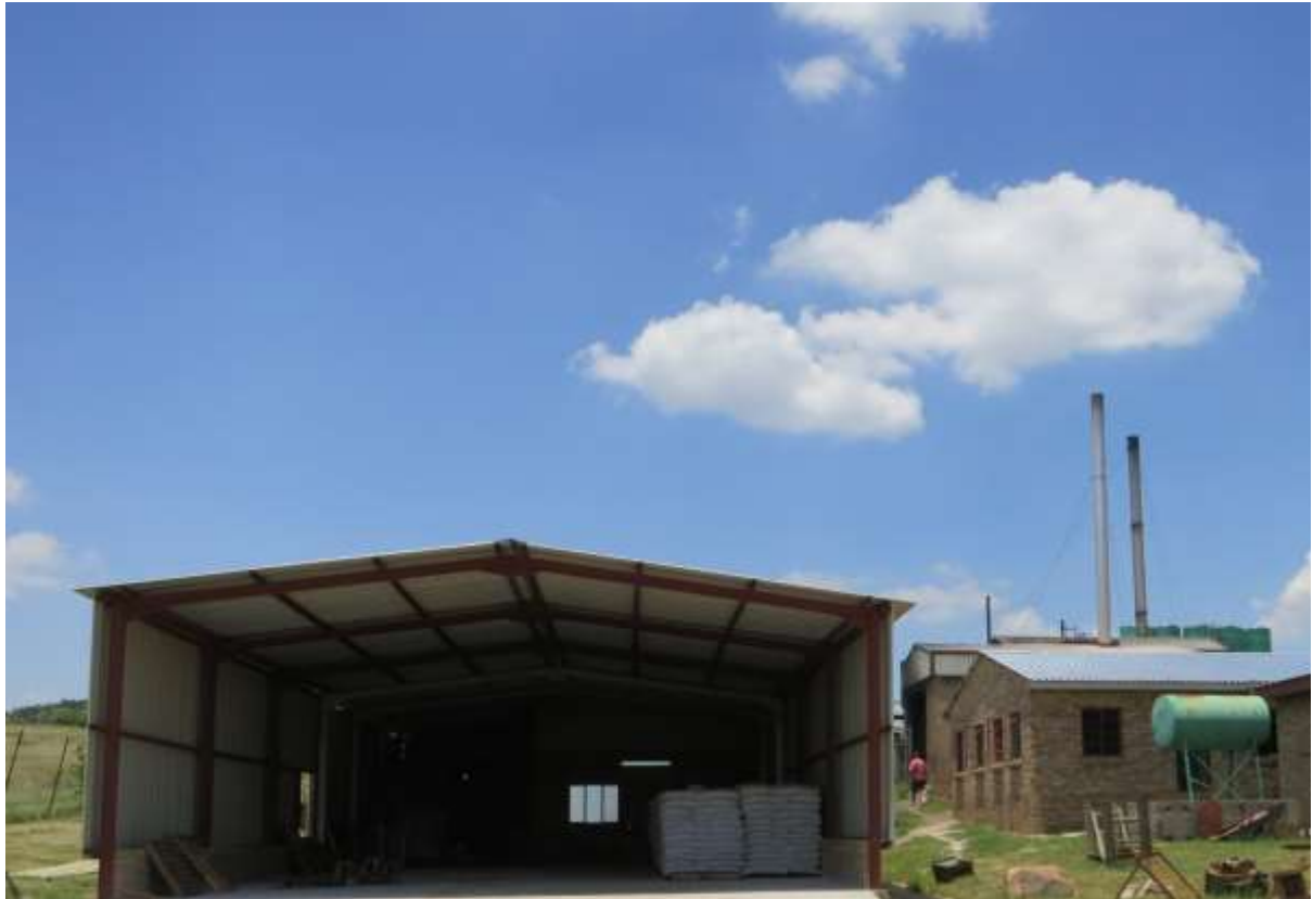
Figure 16: The product storage and dispatch area
