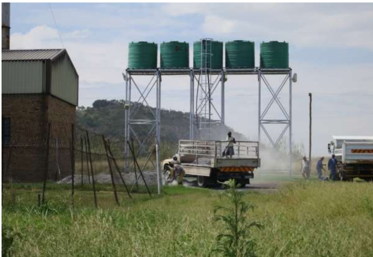
Figure 17: Removal of boiler ash
