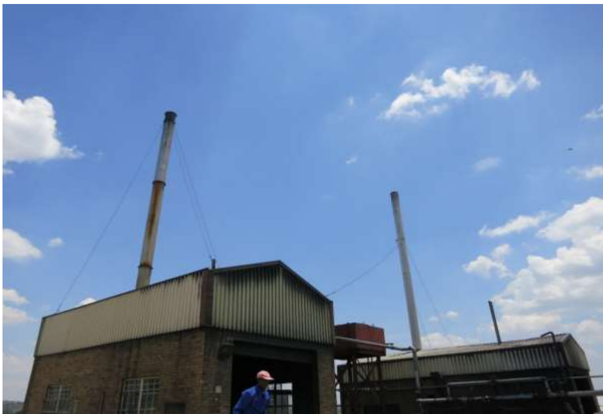
Figure 9: The two boiler stacks
