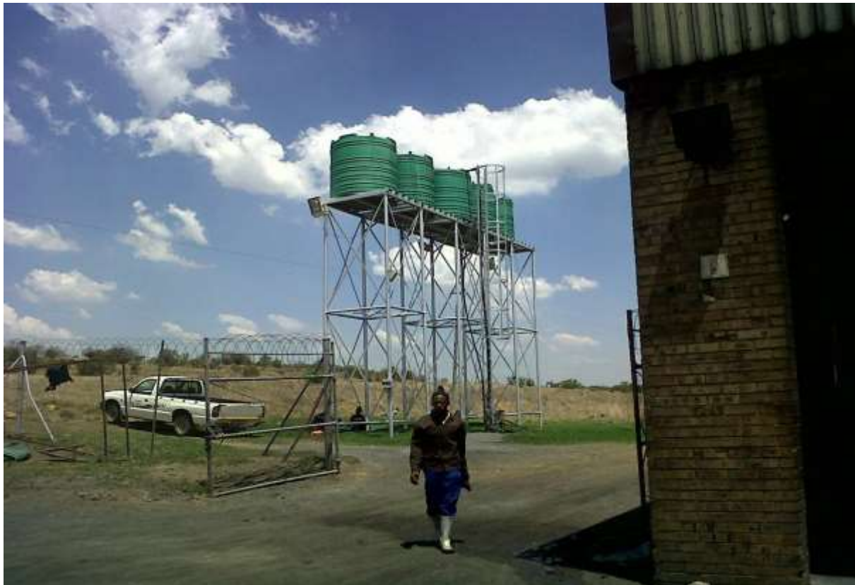
Figure 5: JoJo tanks used to store borehole water from an adjacent property
