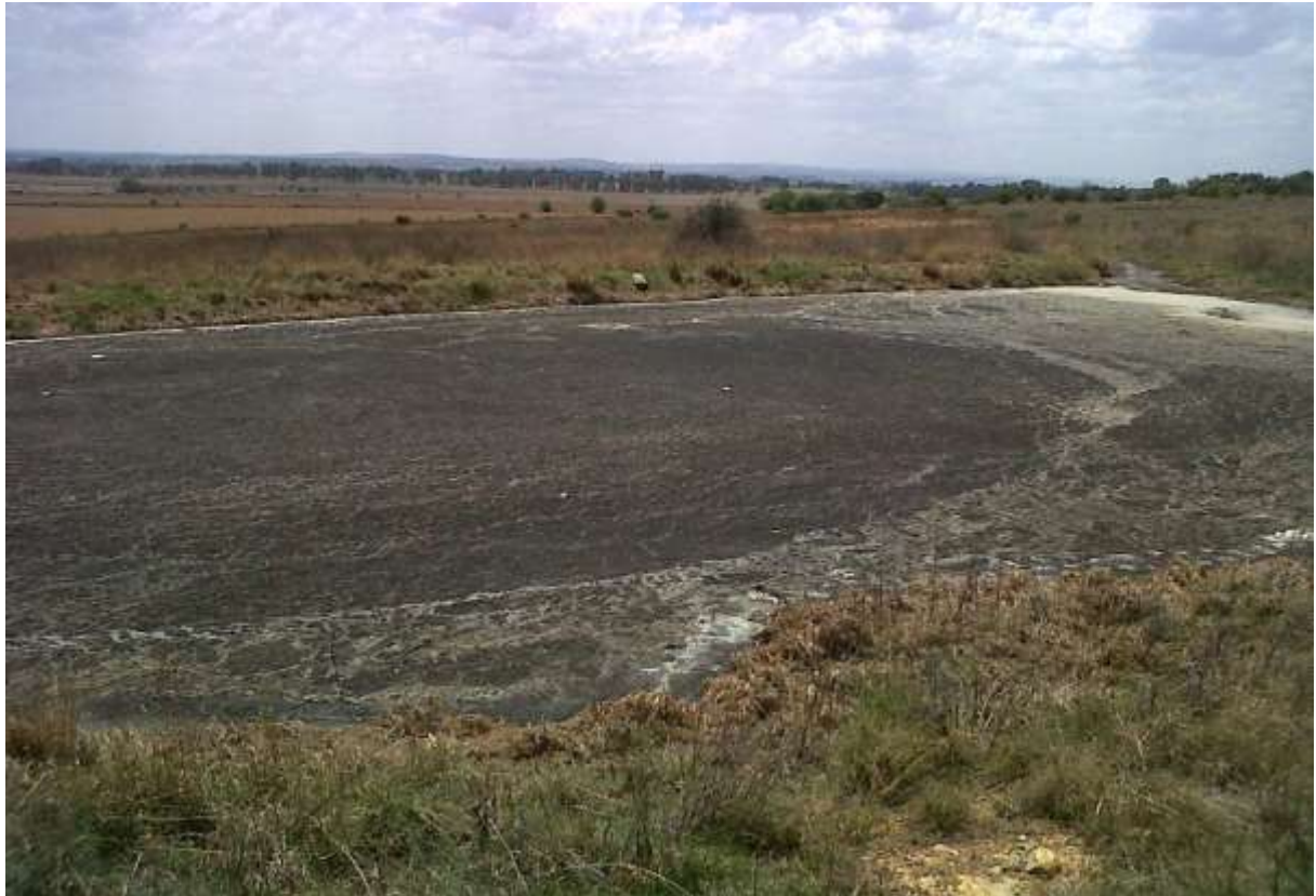
Figure 18: The existing wastewater evaporation pond
