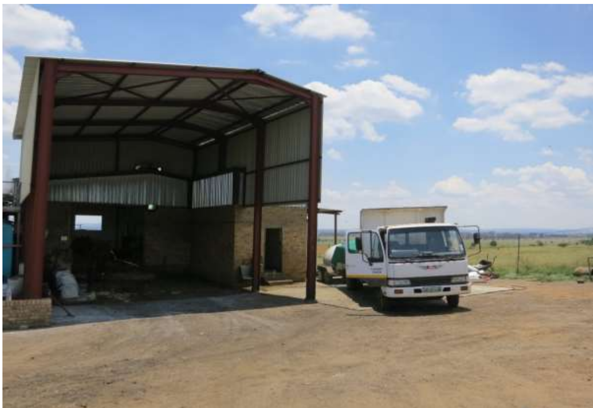
Figure 11: The waste intake area
