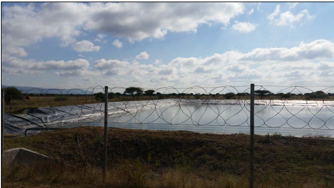
Figure 10: Water retention dam in the southern area of the survey area
