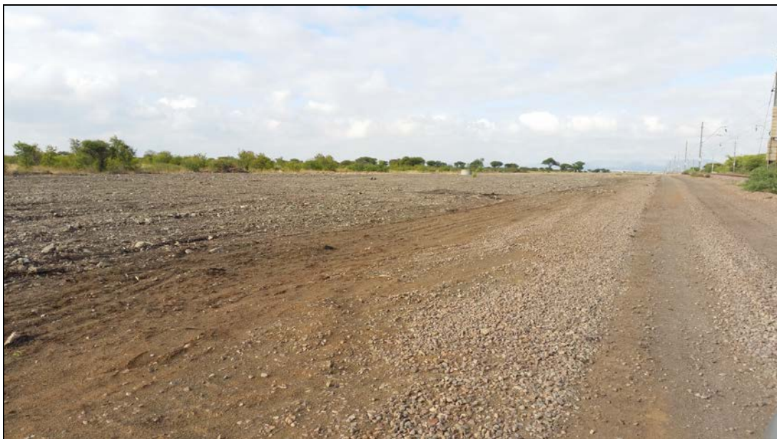
Figure 8: General view of maintenance road along the railway track
