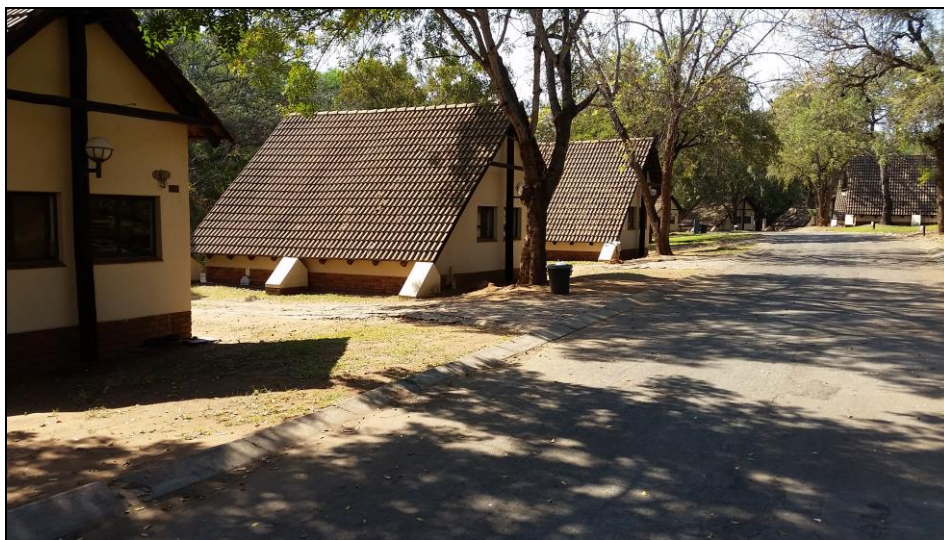
Figure 10: General view of existing infrastructure in the central section of the survey footprint
