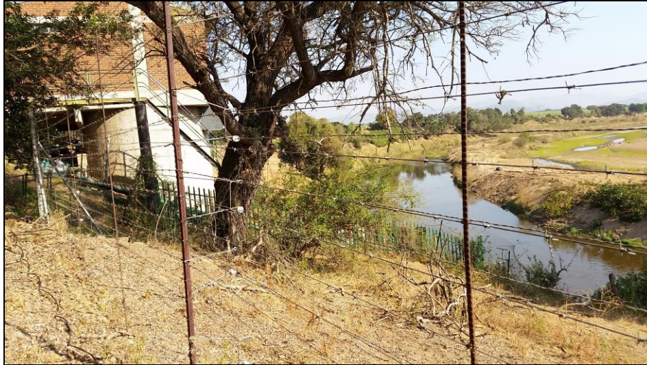
Figure 15: General view of existing infrastructure in the western section of the survey footprint
