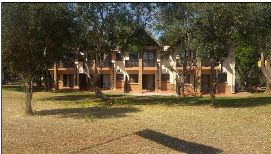
Figure 11: General view of existing infrastructure in the western section of the survey footprint
